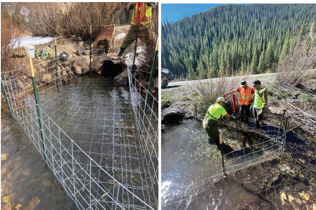
**Figure 2-4:** Highway 550 culvert beaver exclusion fence construction in 2020 (left), and repair work in 2024 (right).
