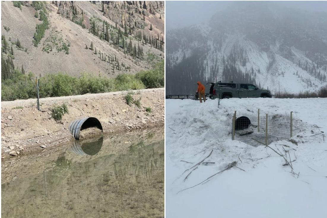
**Figure 2-5.** Country Road 2 culvert beaver damming in summer 2024 (left) and construction of a trapezoidal beaver exclusion fence in December 2024 (right).
