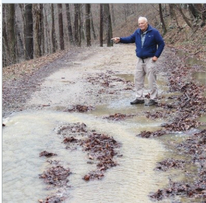
Charlie investigates an eroding area (top) caused by a blocked culvert leading to water pooling on an access road (bottom) used by paddlers. Charlie is part of the FOC Whitewater Access Maintenance Team.
