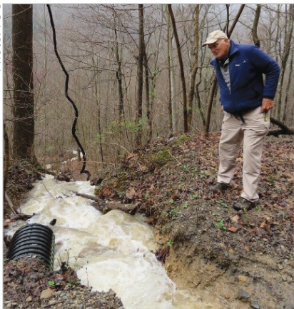
Charlie investigates an eroding area (top) caused by a blocked culvert leading to water pooling on an access road (bottom) used by paddlers. Charlie is part of the FOC Whitewater Access Maintenance Team.
