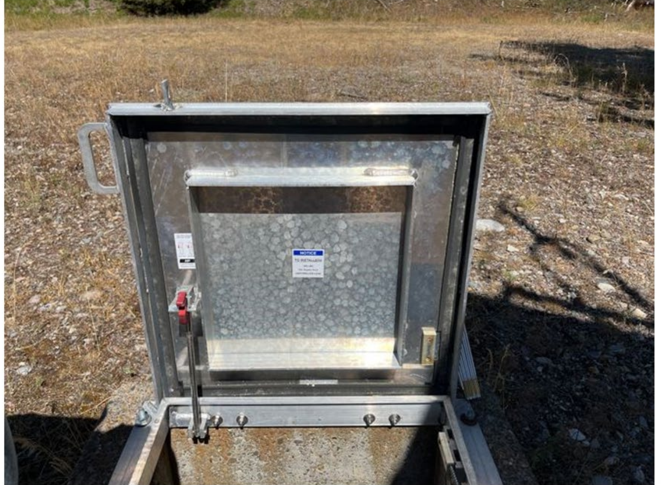
Photo #ST01-4: [REDACTED] - Hatch gasket
