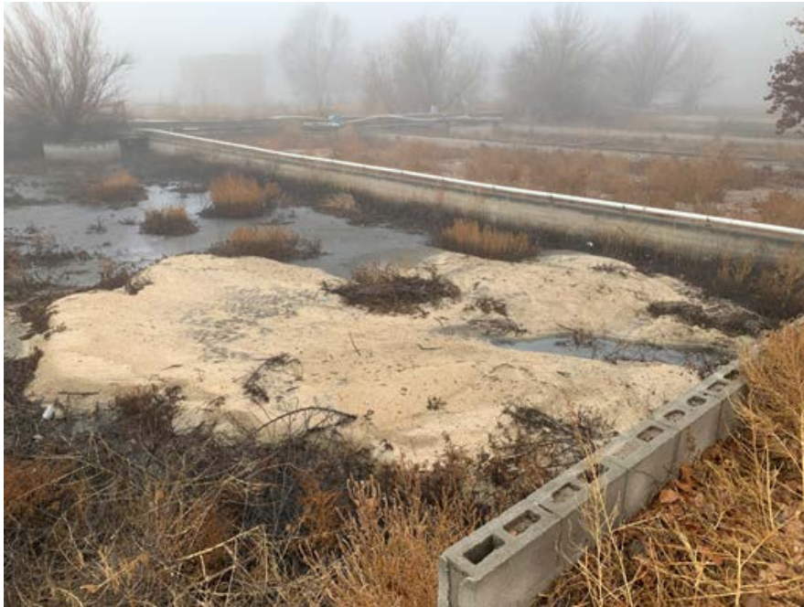
Figure 5.2b - Sediment removed from the UV inlet channel.
