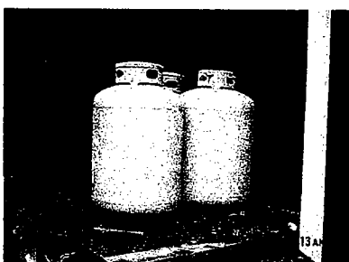
Figure 2-13 (3) Propane Tanks next to Auto Shop.
