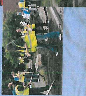
Volunteer students from Exeter High School prepare the soil for the slopes of the rain garden and install the drains and perennials.
