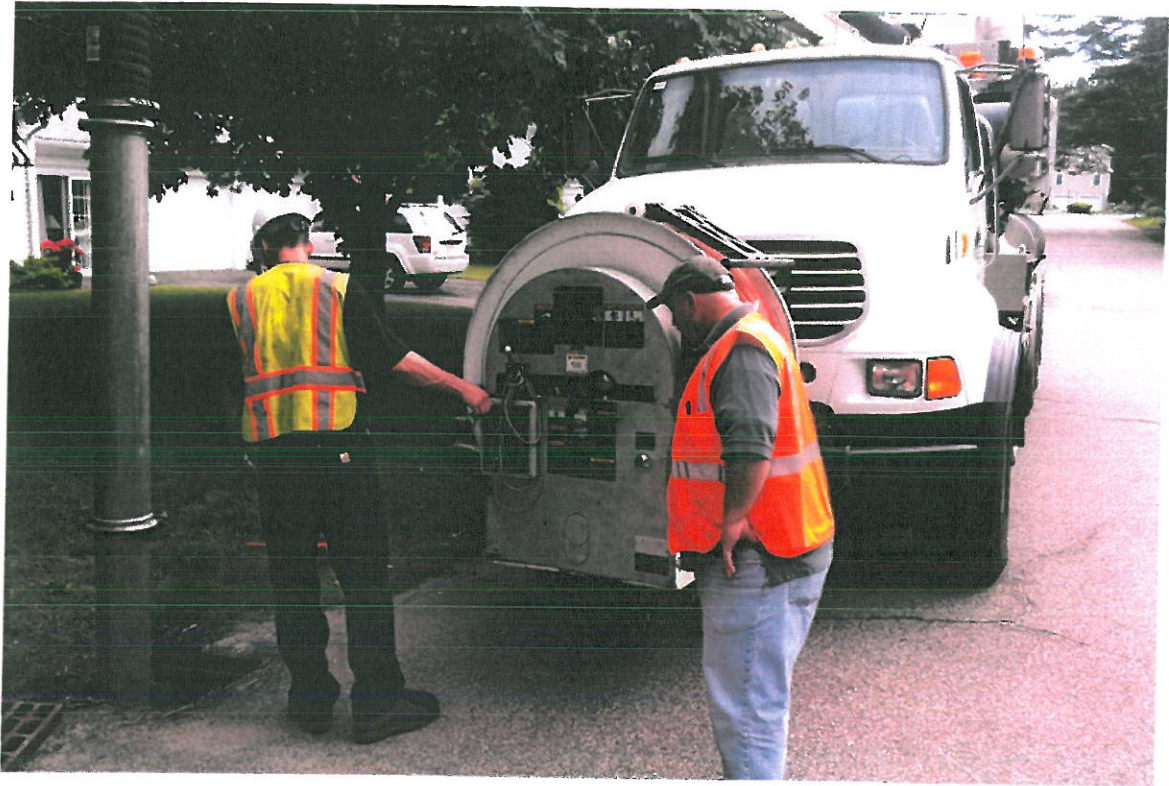
CLEANING CATCH BASINS
