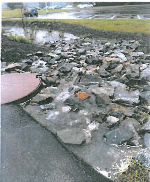
This bioretention unit is an example of a stormwater management activity that would be tracked and credited.
