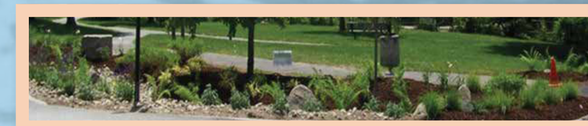
The Exeter Department of Public Works prepares the rain garden under the design and direction of Ironwood design group. Boulders slow water as it enters the garden off the steep hill of Chestnut Street. A special compost mix quickly infiltrates the stormwater back into the groundwater table.
