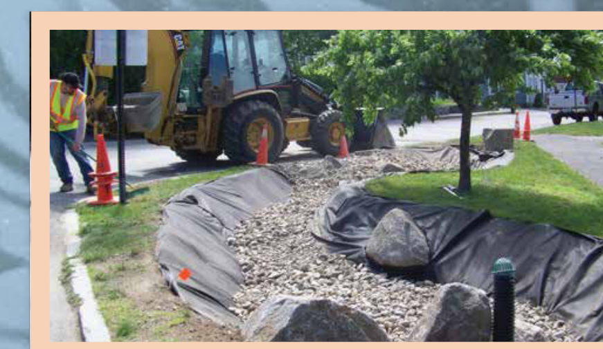
The Exeter Department of Public Works prepares the rain garden under the design and direction of Ironwood design group. Boulders slow water as it enters the garden off the steep hill of Chestnut Street. A special compost mix quickly infiltrates the stormwater back into the groundwater table.
