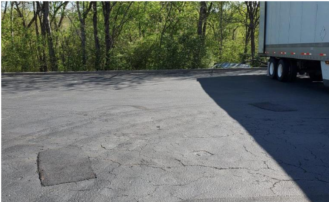
Asphalt Repair 2: Eastern portion of Asphalt Cap facing East. Additional examples of repairs to the asphalt.
