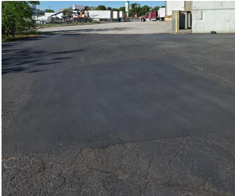
Asphalt Repair 1: Southern boundary of Asphalt Cap facing Southwest. Repairs were made in an area of asphalt surface deterioration noted in 2024 annual report.
