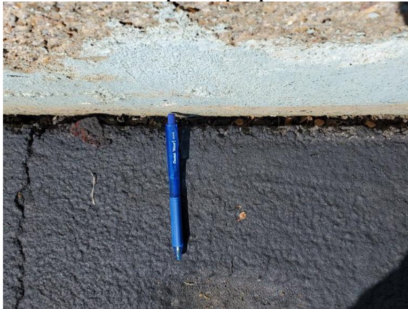
At eastern side of building facing West. A gap between the building and asphalt cap has been reported since the 2018 Annual Inspection and Cap Maintenance Report. Gap does not appear to have increased significantly.
