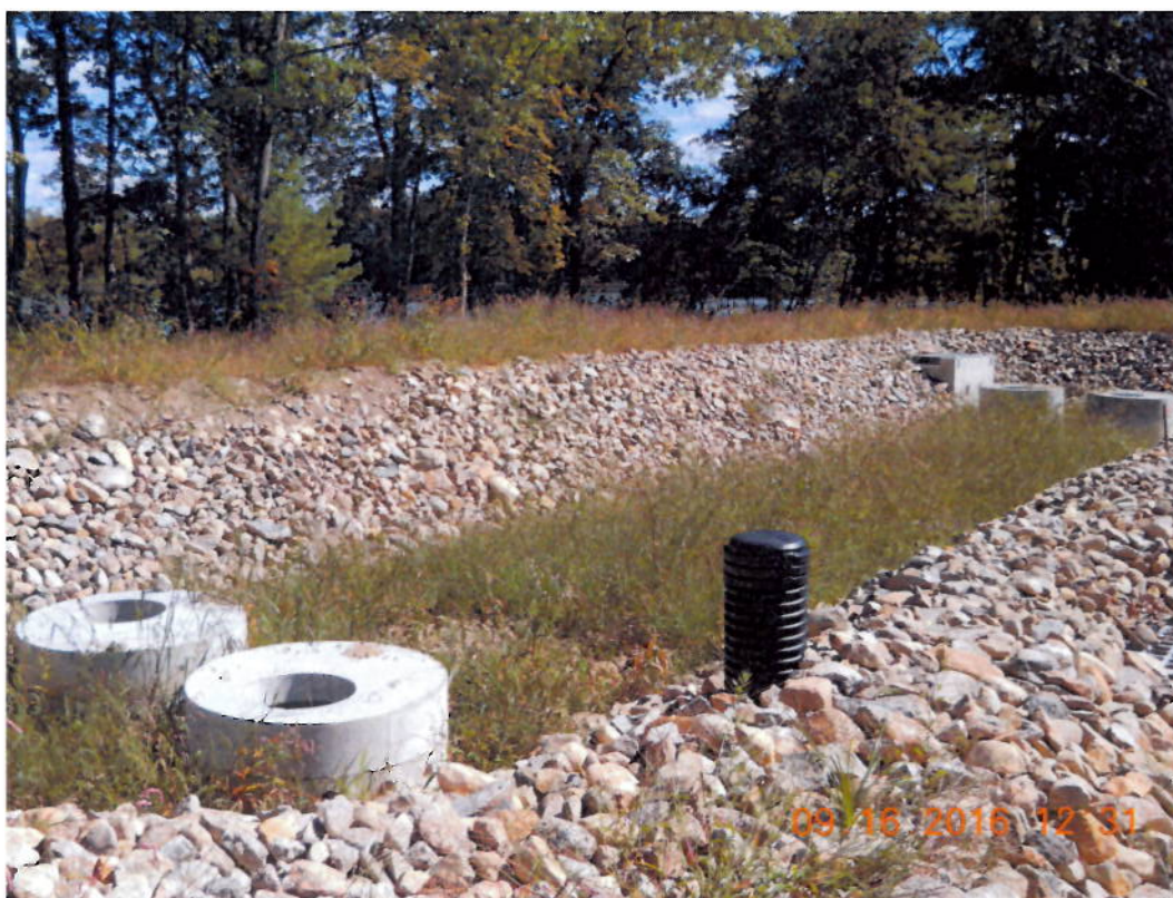
Gravel Wetland Cell at Nutt Pond
