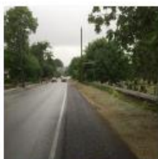
Sagamore Ave. Reconstruction with Porous Pavement
