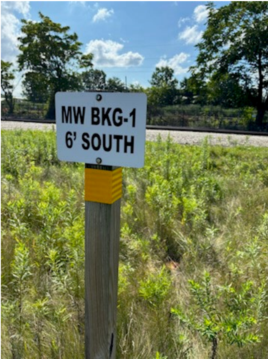
Picture 2: SWMU 5 monitoring well MW BKG-1 and signage
