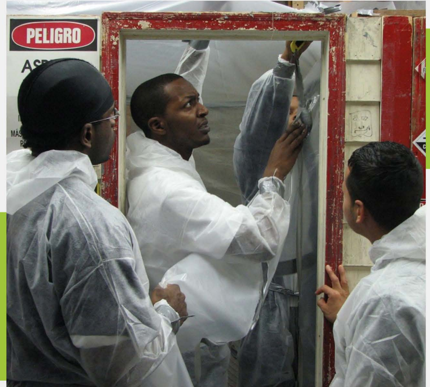
Students in technical training sealing doorway - St. Nicks Alliance, Brooklyn, NY
