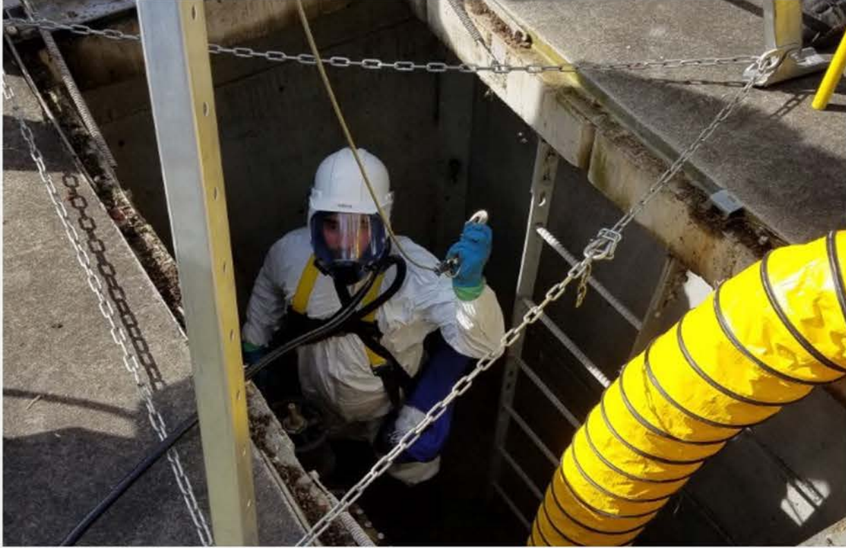
Practicing underground storage tank tasks - City of Tacoma, WA
