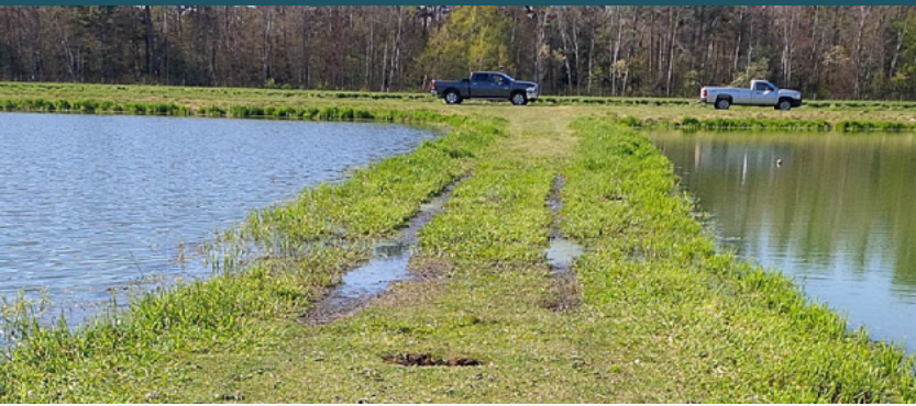
The previous wastewater treatment lagoon had high water seepage (above), necessitating improvements to the system to protect natural resources. Below, a new forcemain is installed from the new lift station to the MBBR wastewater treatment facility.
