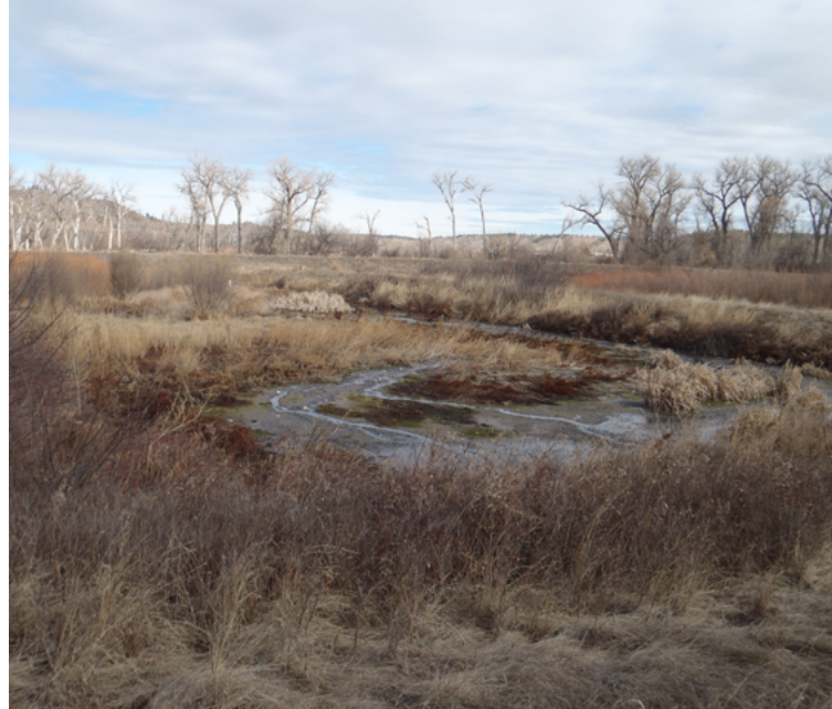
The renovation cleared the vegetation from the lagoon, resealing this cell and constructing another.
