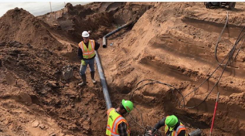
The previous wastewater treatment lagoon had high water seepage (above), necessitating improvements to the system to protect natural resources. Below, a new forcemain is installed from the new lift station to the MBBR wastewater treatment facility.
