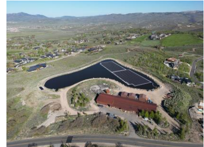
Photo credit: Mountain Regional Water Special Service District
