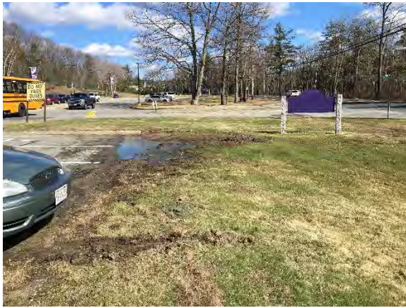
Figure 4. Rain Garden Site
