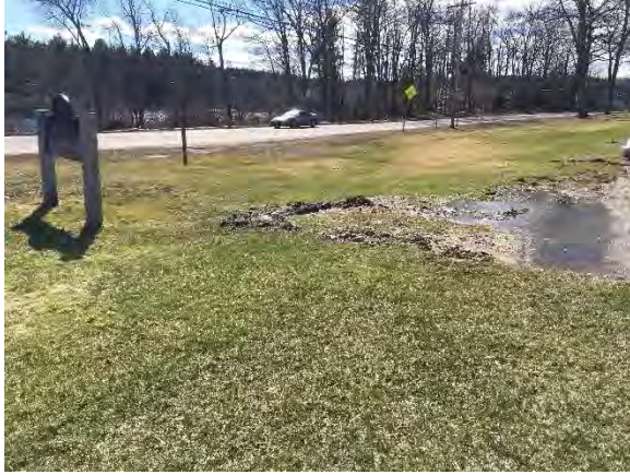
Figure 2. Rain Garden Site
