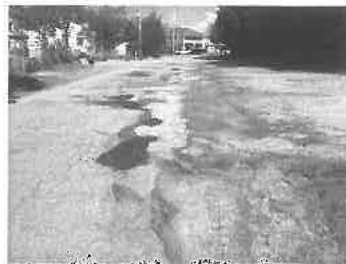
Bay Ave East - Pavement Damaged - Puddling - Slow Drainage
