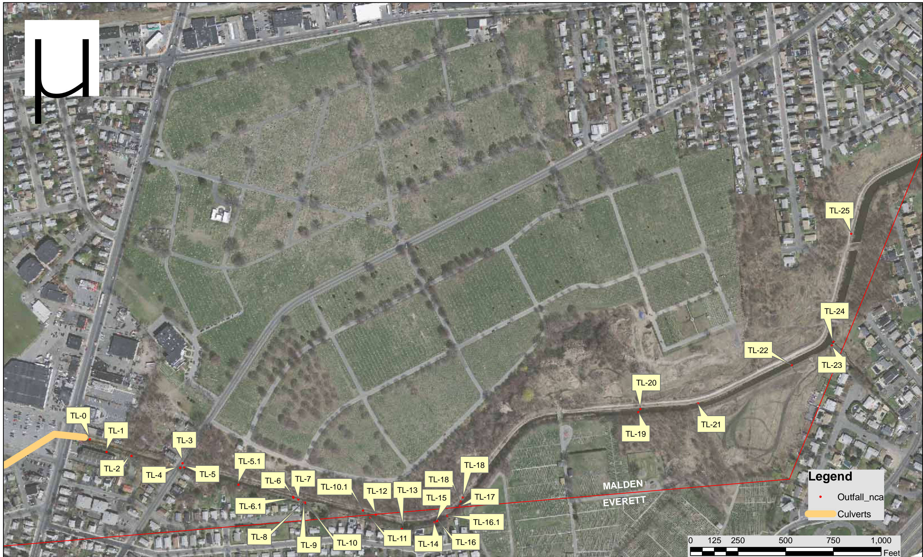
Figure 7 - Town Line Brook Outfalls (updated 11-10-11)
