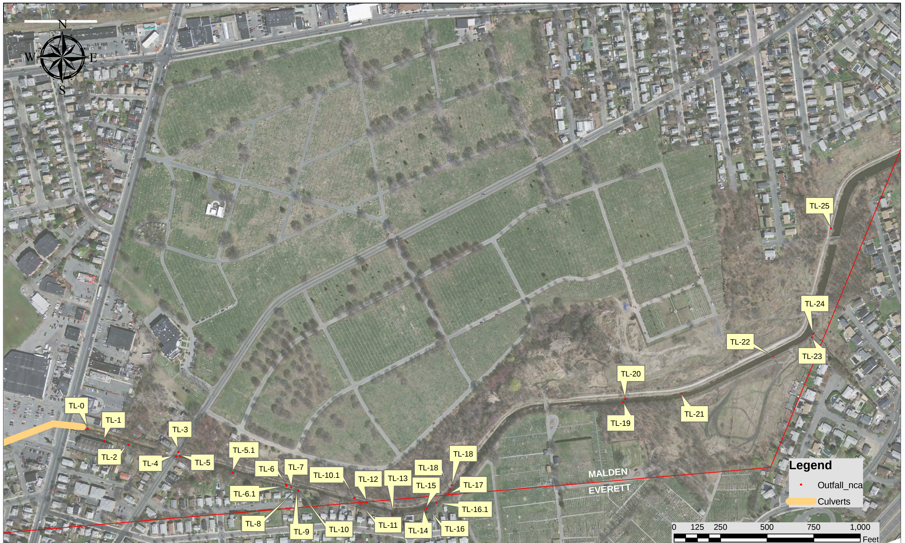
Figure 3 - Town Line Brook Outfalls
