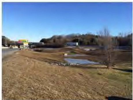
Weston Tolls – Wet Pond construction complete
