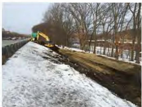
Boston- I-90 Westbound- Infiltration Basin construction
