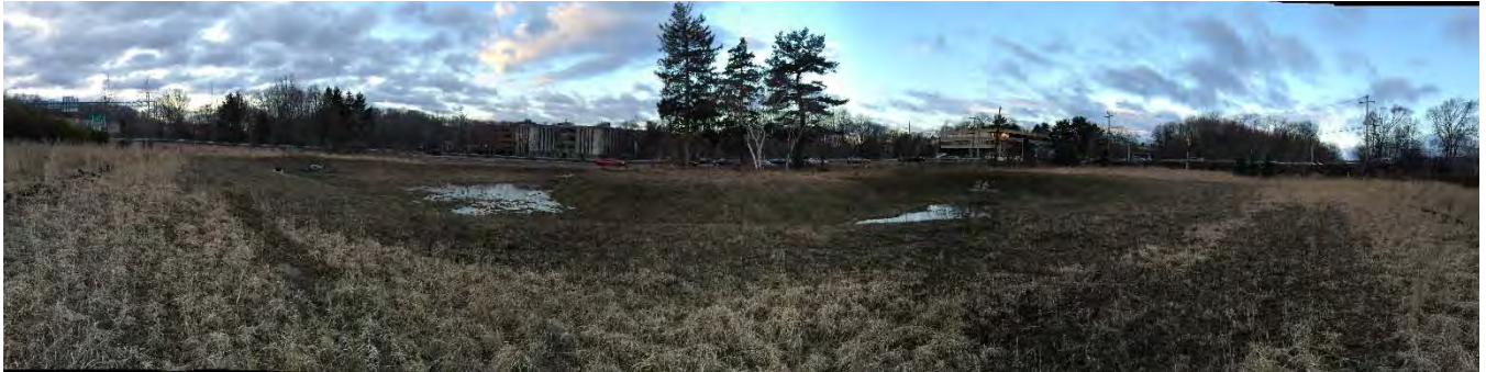
Photo 1. BMP 13, Infiltration Basin – Looking West
