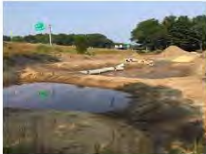
A roadside pond is being constructed next to Route 2 West by Exit 52A to collect and treat stormwater runoff.
