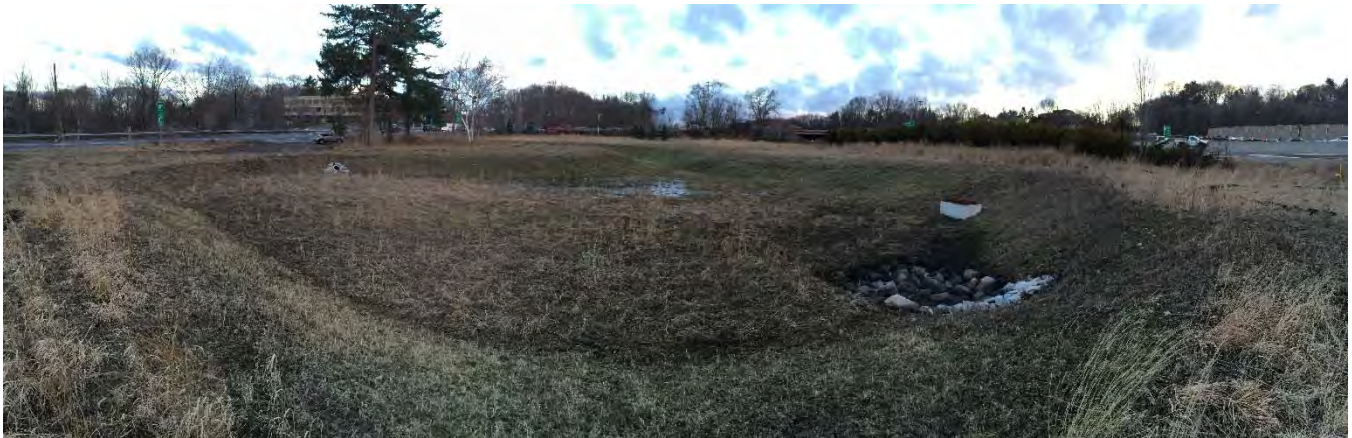
Photo 2. BMP 13, Infiltration Basin – Looking North
