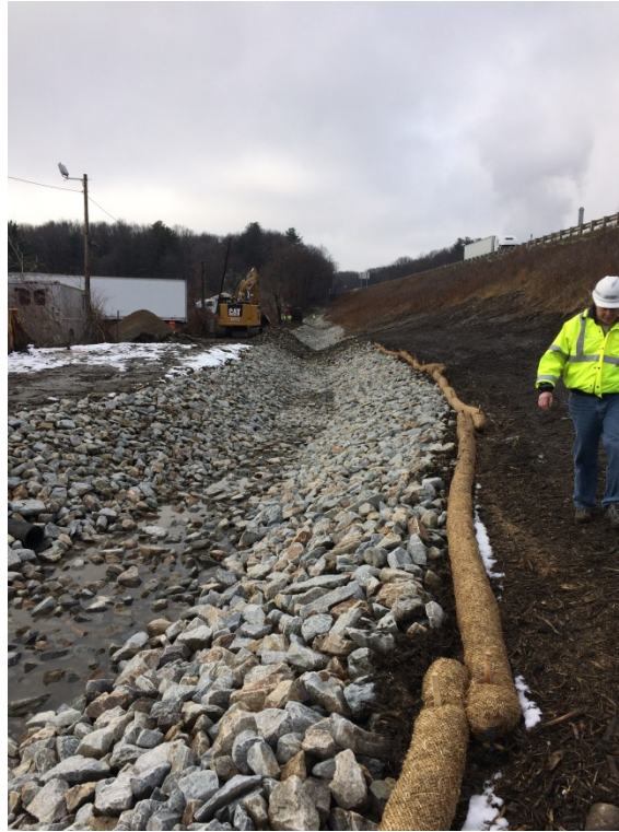
Photo 1. Constructed Infiltration Swale
