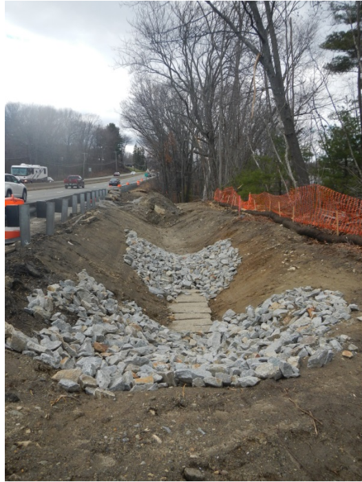
Photo 1. Constructed Infiltration Swale
