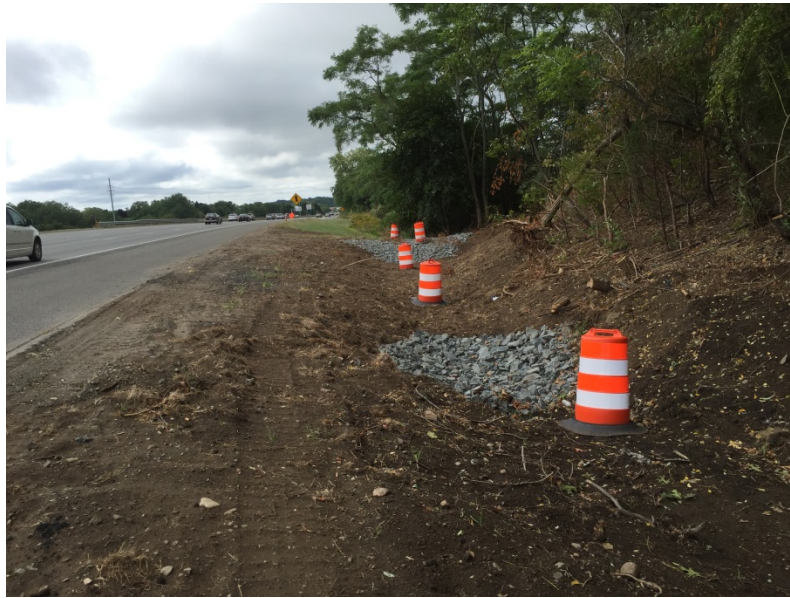
Photo 1. Construction of an Infiltration Swale
