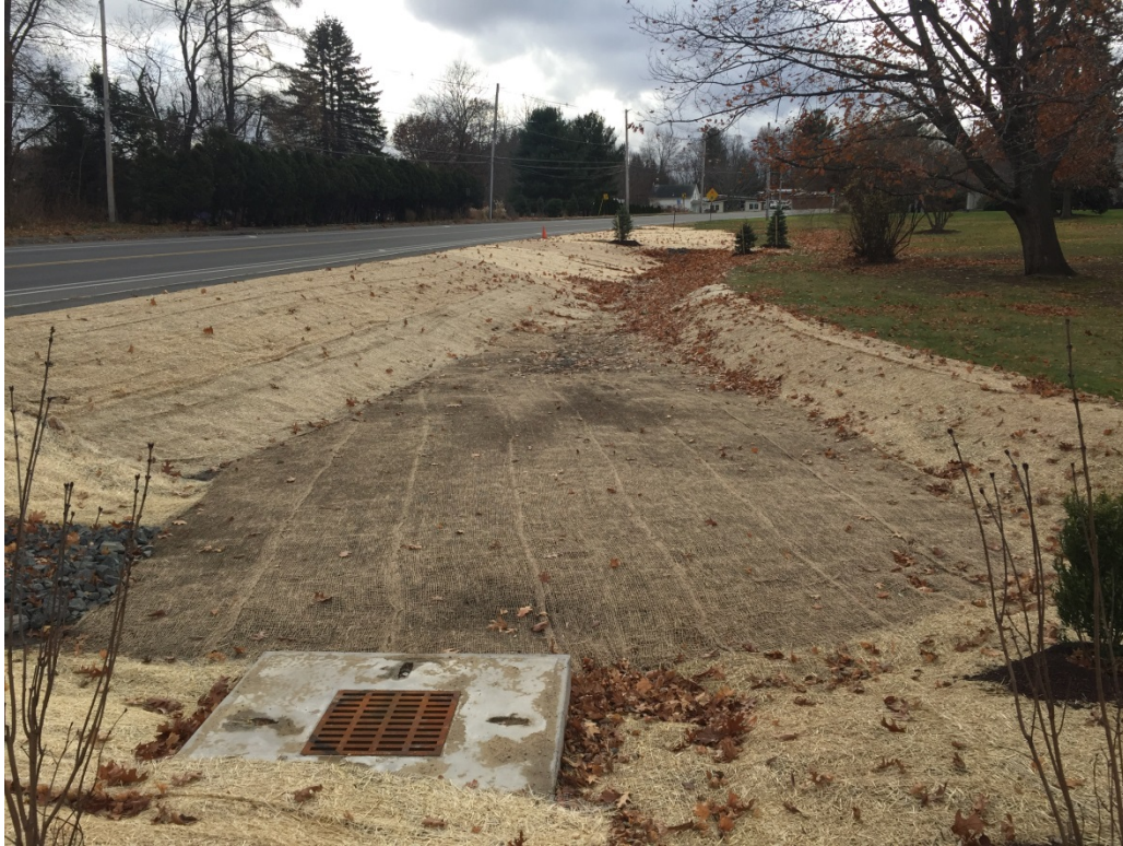
Photo 1: Stormwater BMP looking south from Route 116.
