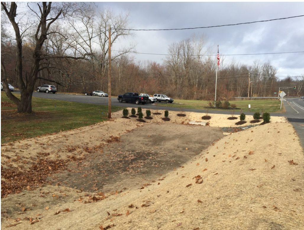
Photo 2: Stormwater BMP looking north from Route 116.
