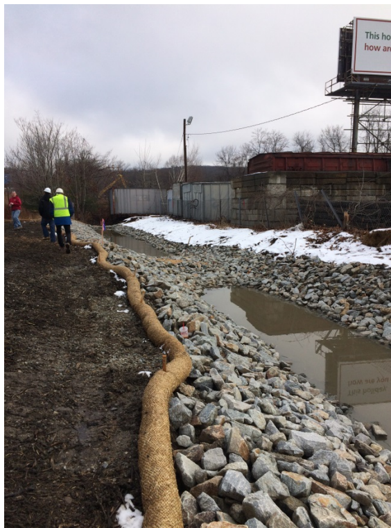
Photo 2. Constructed Infiltration Swale
