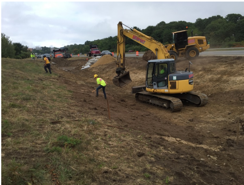
Photo 2. Construction of an Infiltration Swale
