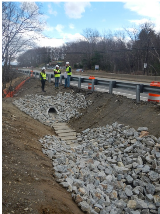
Photo 2. Constructed Infiltration Swale
