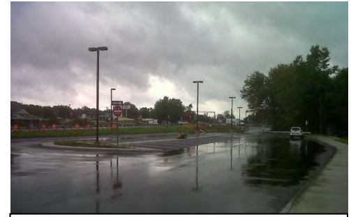
Permeable Pavement Parking Lot
