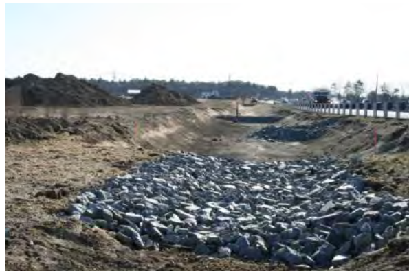
Construction of Infiltration Basin
