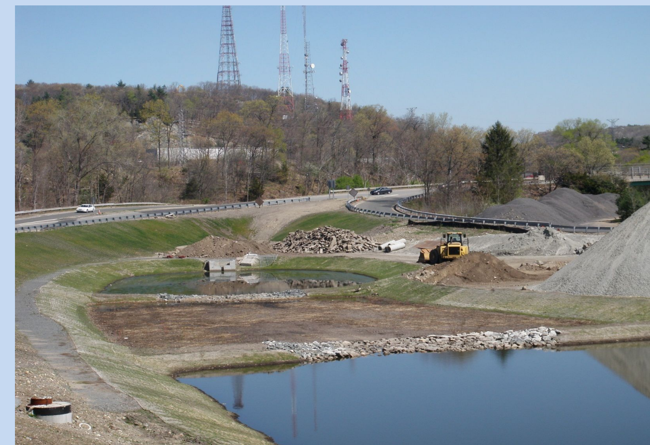
Gravel wetland with wet ponds under construction along Rt. 128 at outfall WA-17
