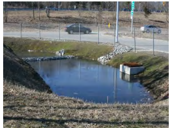
Construction of Dry Detention Basin
