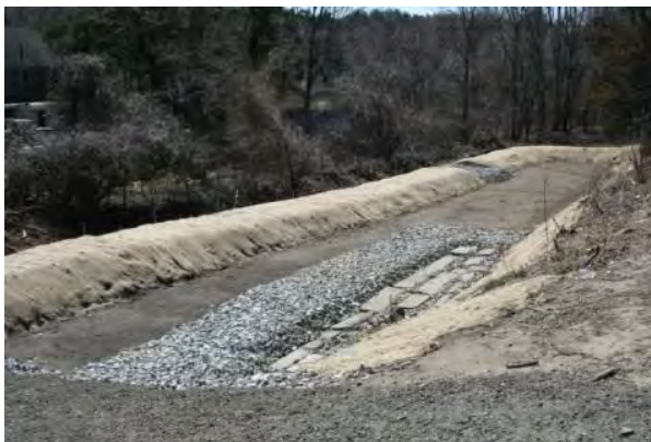
Construction of Infiltration Basin
