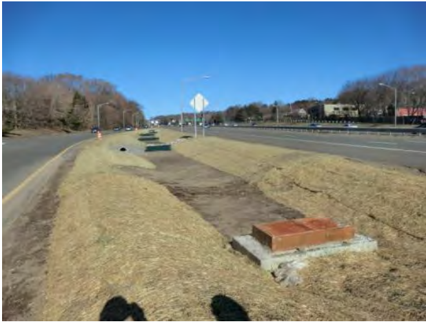
Construction of Infiltration Basin
