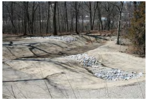
Construction of Infiltration Basin
