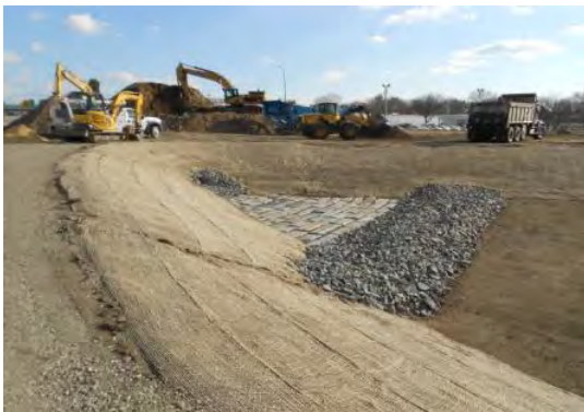
Construction of Infiltration Basin
