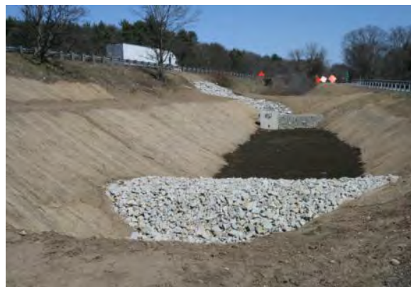
Construction of Infiltration Basin
