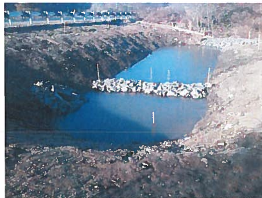
Construction of Infiltration Basin
