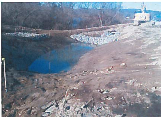
Construction of Infiltration Basin
