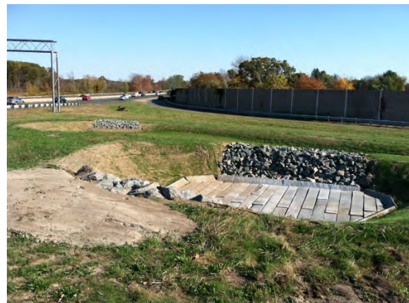
Construction of Infiltration Basin Forebay
