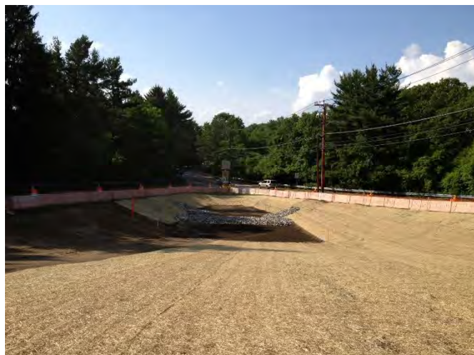
Construction of Recharge Basin #1
