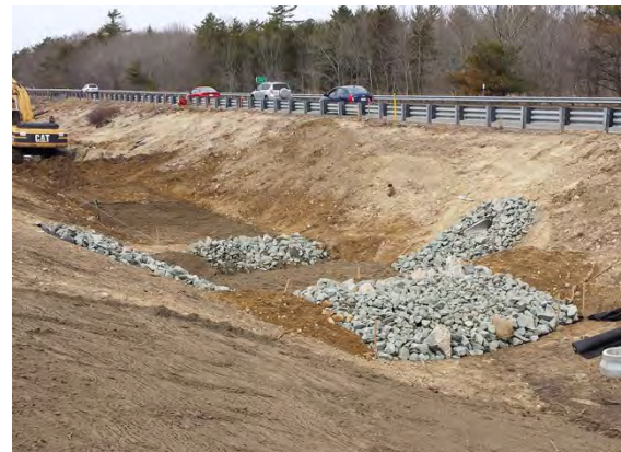
Construction of Infiltration Basin Forebay
