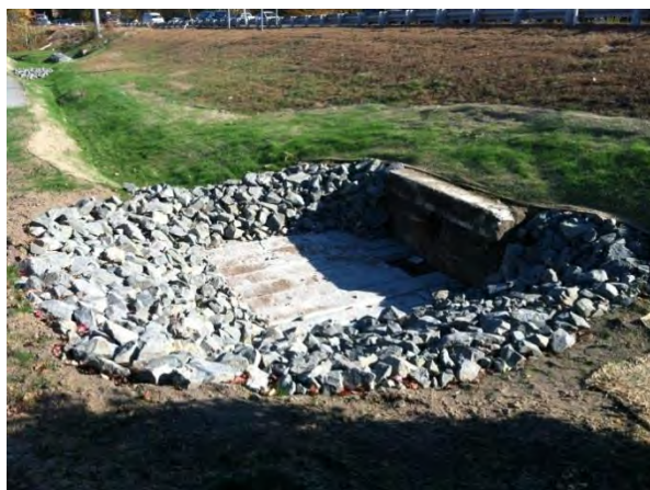
Construction of Infiltration Basin Forebay
