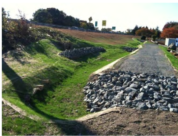
Construction of Infiltration Basin
