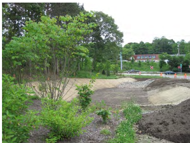
Construction of Recharge Basin #2
