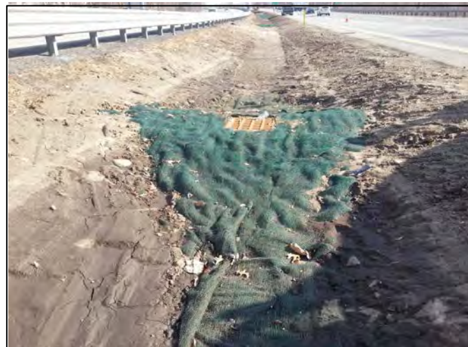
Infiltration swale in I-290 Median
