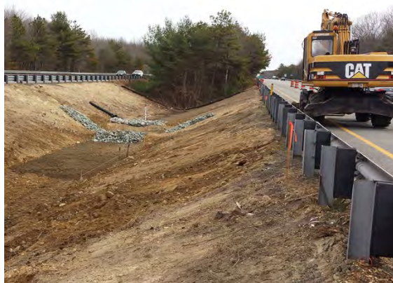
Construction of Infiltration Basin
