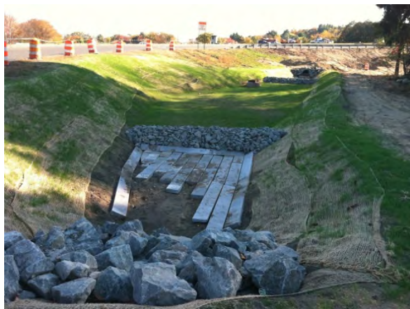
Construction of Infiltration Basin
