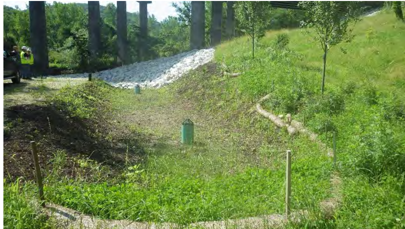
Completed Gravel Wetland
