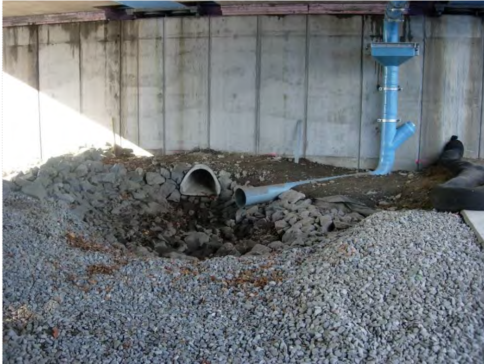
Sediment Forebay for Constructed Infiltration Basin
