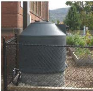
Cistern - Center Pepin Elementary School, Easthampton
