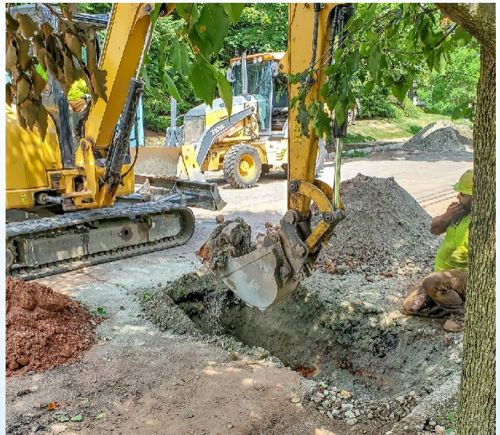
In search of lead service lines.
