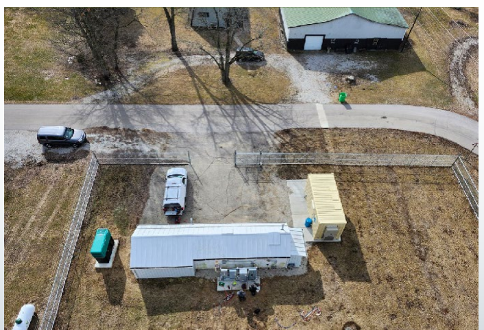
Overhead view of the plant.
