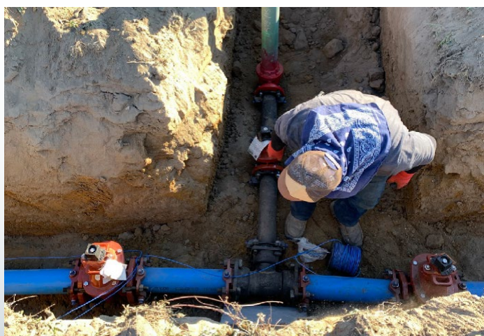
Installation of water main and post hydrant.
