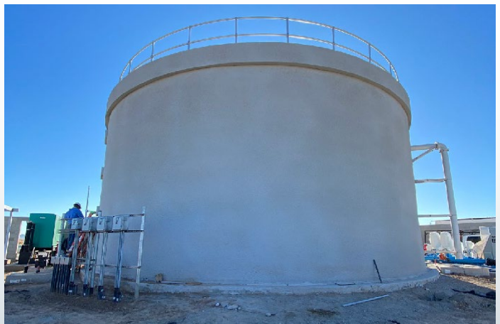
Completed water storage tank.
