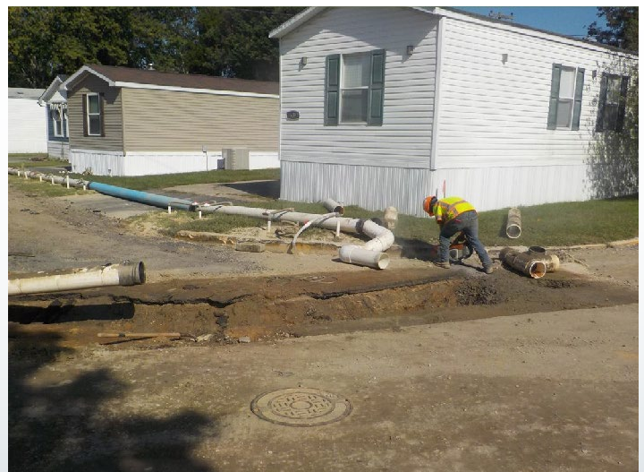
Workers on site positioning and laying down water distribution piping.
