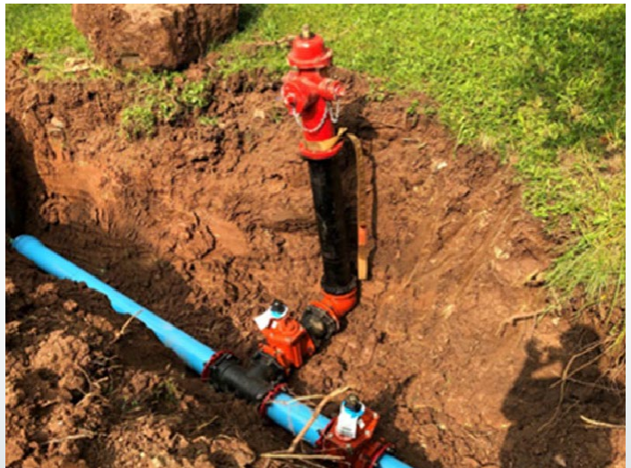
Fire hydrant installation on Fish Hatchery Road.
