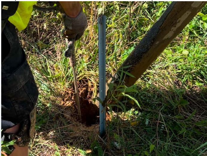
Hillsville crew excavating service line to identify material.
