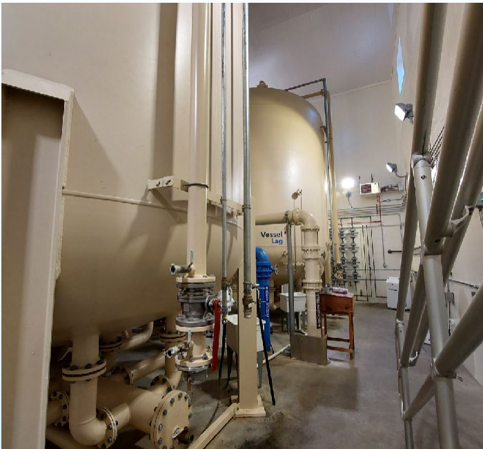
Merrimack Village District water treatment plant construction site.
