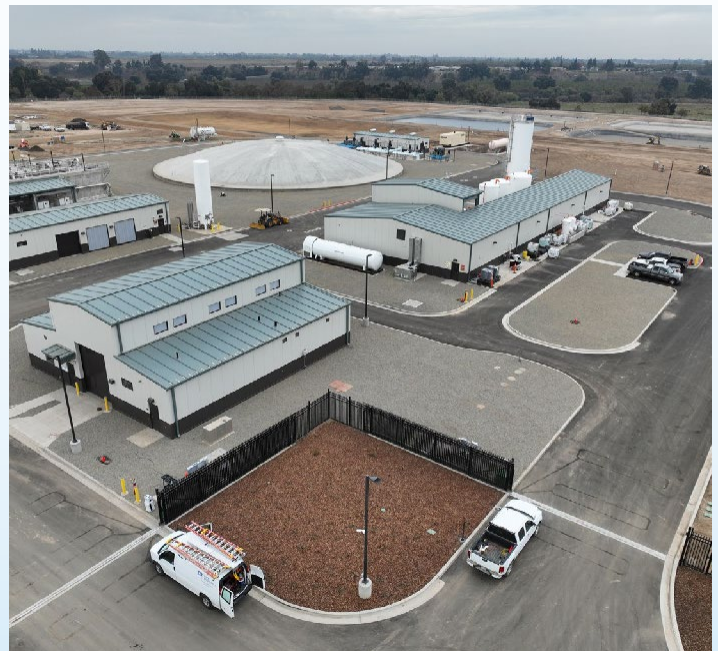
Aerial view of the water treatment plant.
