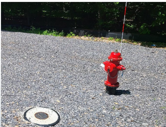
Newly installed fire hydrant and municipal casting.
