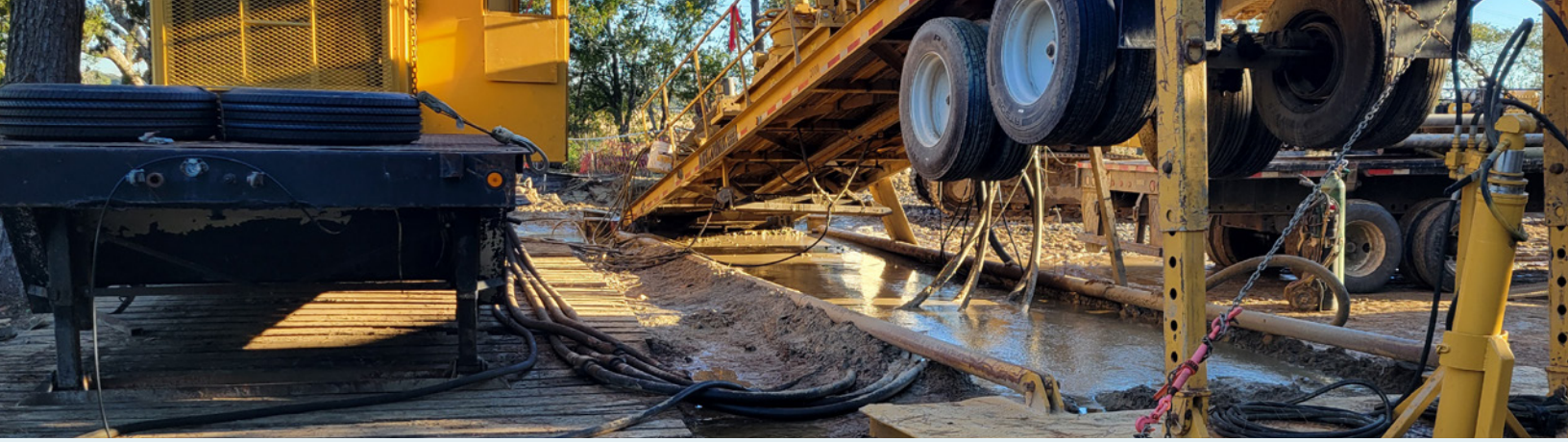
Photo credit: James Island Public Service District (JIPSD)
