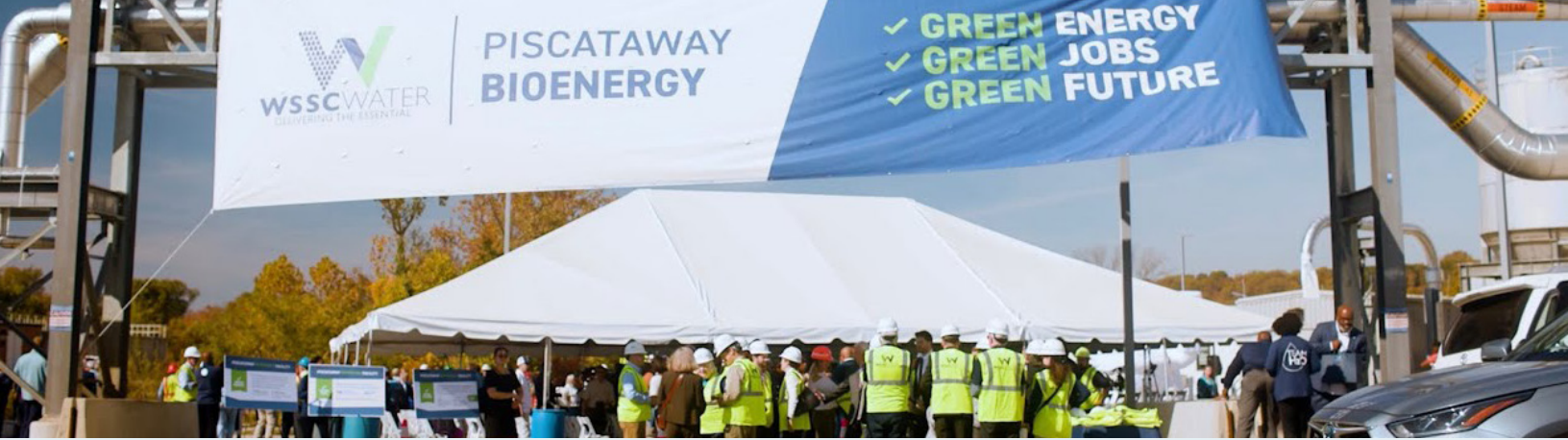
Photo credit: Washington Suburban Sanitary Commission (WSSC)
