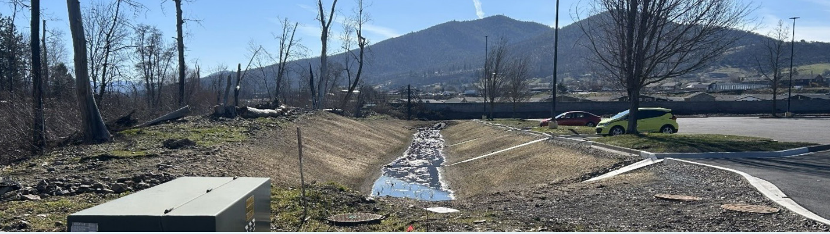
Photo credit: Rogue Valley Sewer Services
