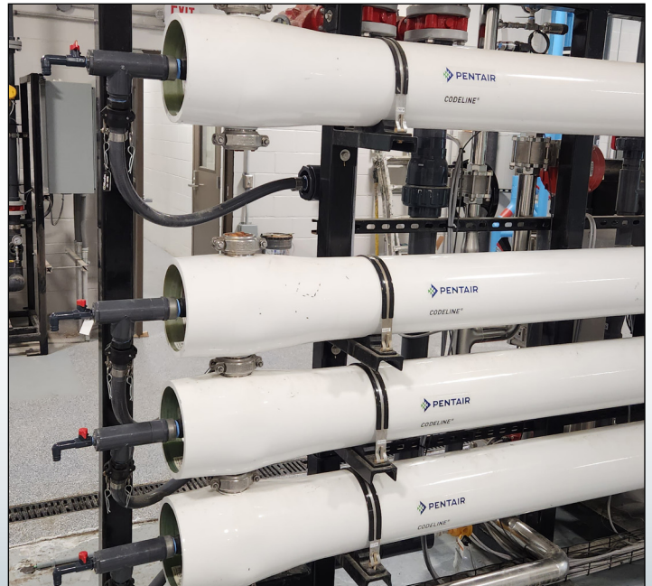
Reverse osmosis filters used to remove contaminants from drinking water.
