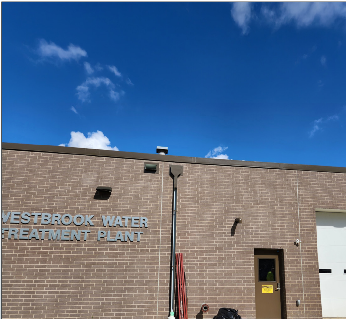
New water treatment plant.
