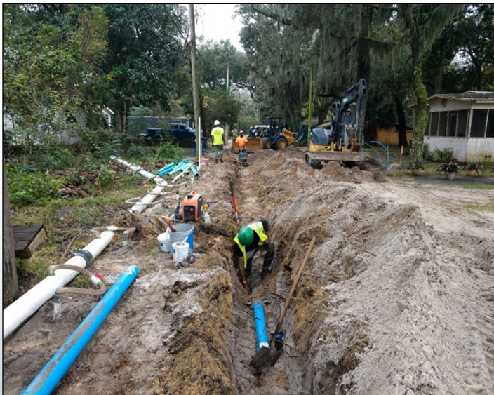
Water main installation on Leonard Street.
