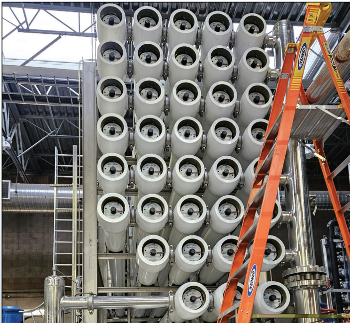
Construction of the desalination plant's reverse osmosis train.
