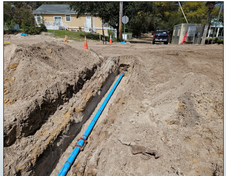
Water main installation on James Street.
