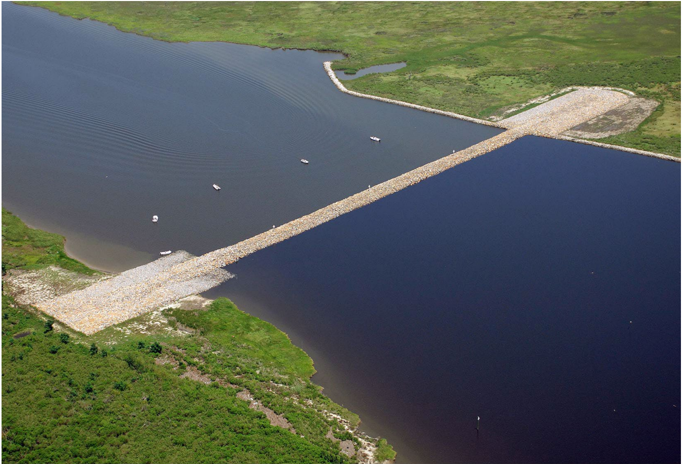
3631 3632 Figure 47. Closure structure across MRGO completed in 2009.
