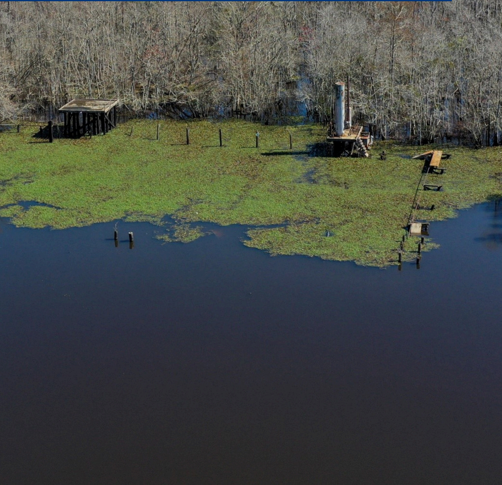
Oil and gas infrastructure near Lake Maurepas in St. John the Baptist Parish (Photo Credit: CPRA).
