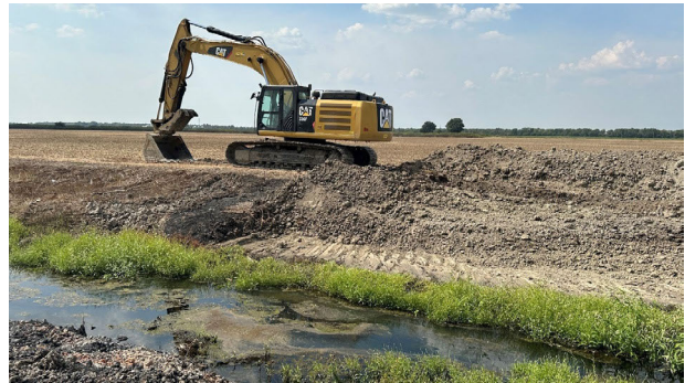
Before and during two-stage ditch construction near Delaplaine, Arkansas. Banks were vegetated with winter oats and brassica
