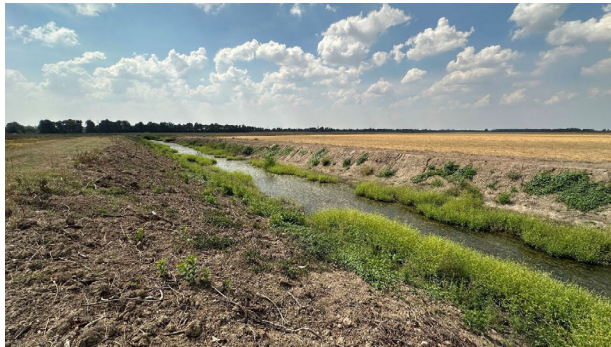
Before and during two-stage ditch construction near Delaplaine, Arkansas. Banks were vegetated with winter oats and brassica
