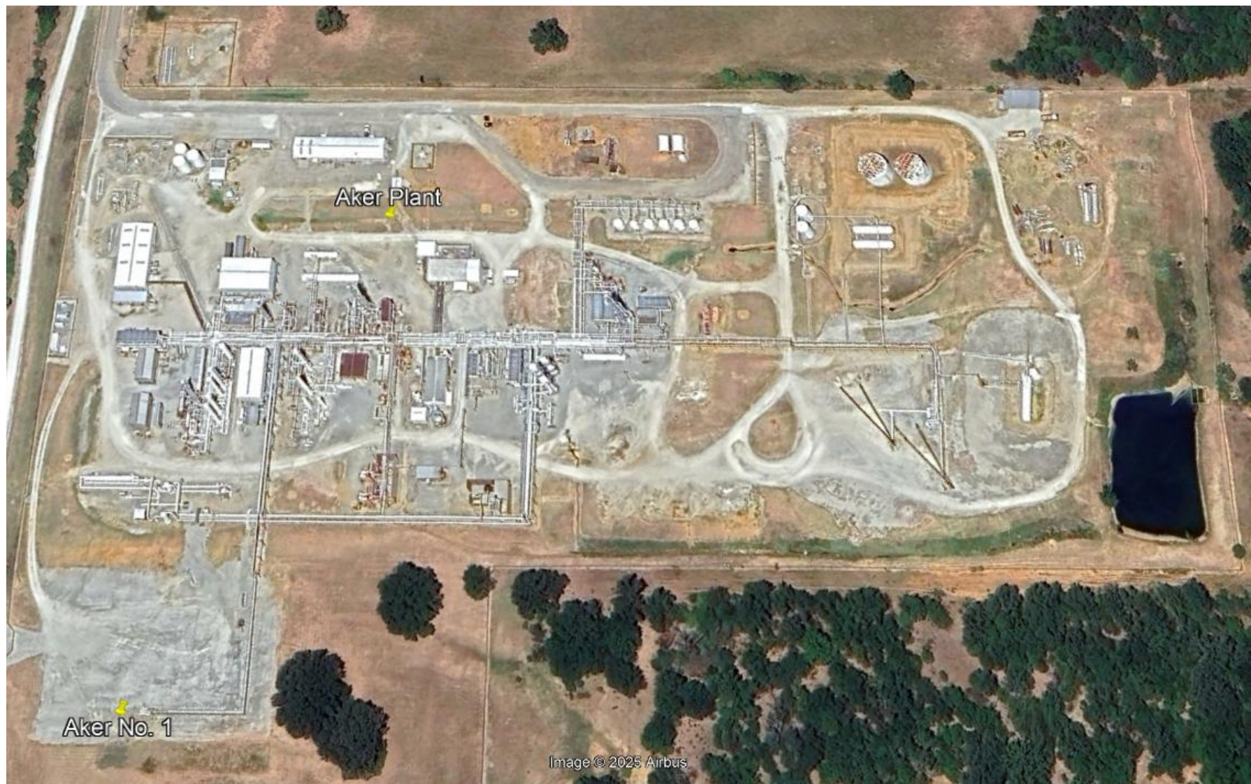
Figure 2 – Aker Plant and Aker Gas Injection No. 1.
