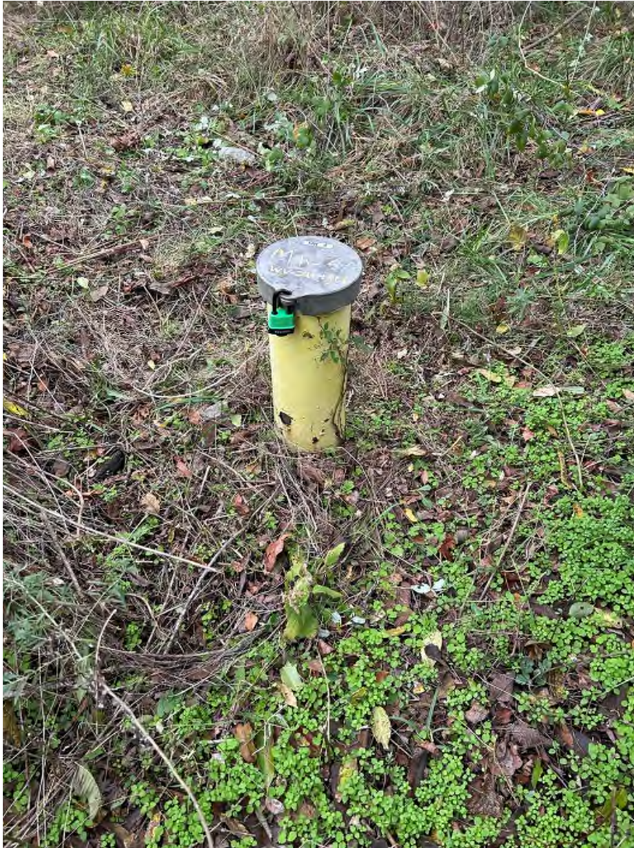
Figure 6: Image of the well MW-4 as seen during the site walk.
