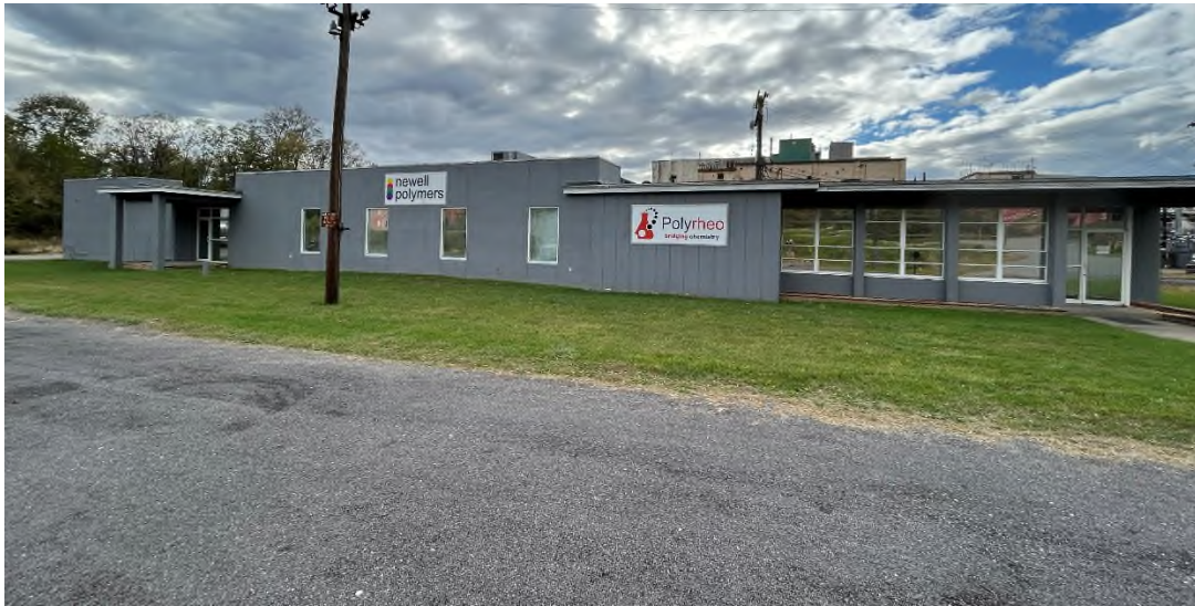
Figure 3: Main office building of the facility as seen from the car parking lot.
