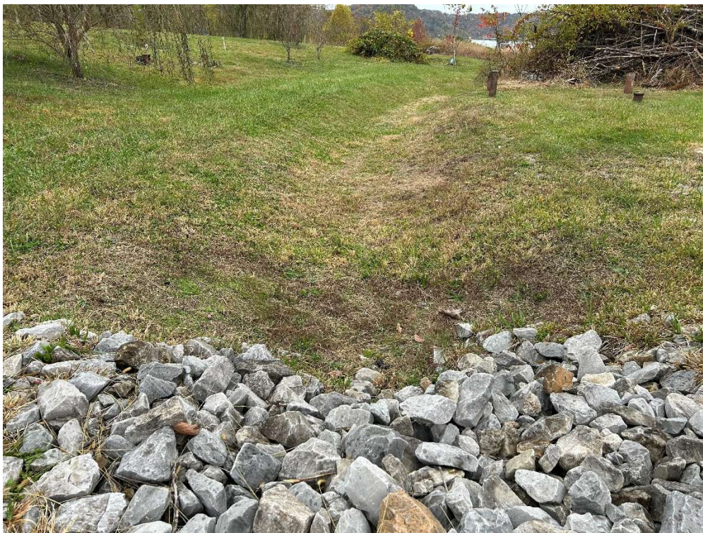
Image 7: Looking toward the swale from the edge of the drainage improvement area with riprap covering piping
