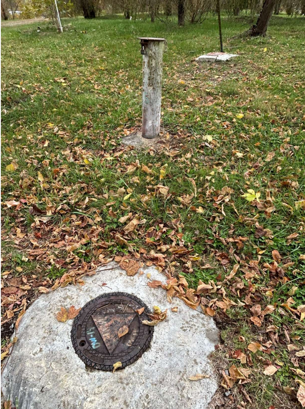
Image 10: A cluster of three monitoring wells (DW-14, M-35, and MW-41) in the southeastern corner of Area 7
