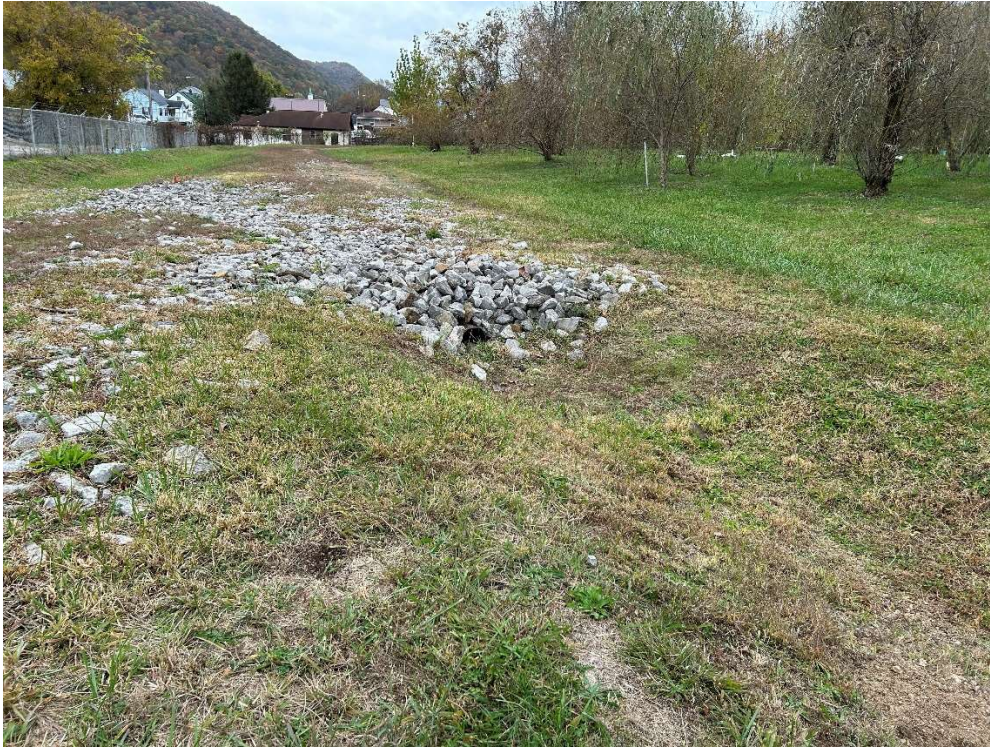
Image 7: Looking toward the swale from the edge of the drainage improvement area with riprap covering piping
