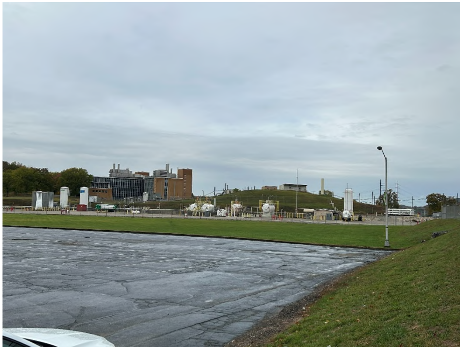
Figure 5: Lower Ward Landfill. Looking west. An empty portion of the parking lot/landfill cover.
