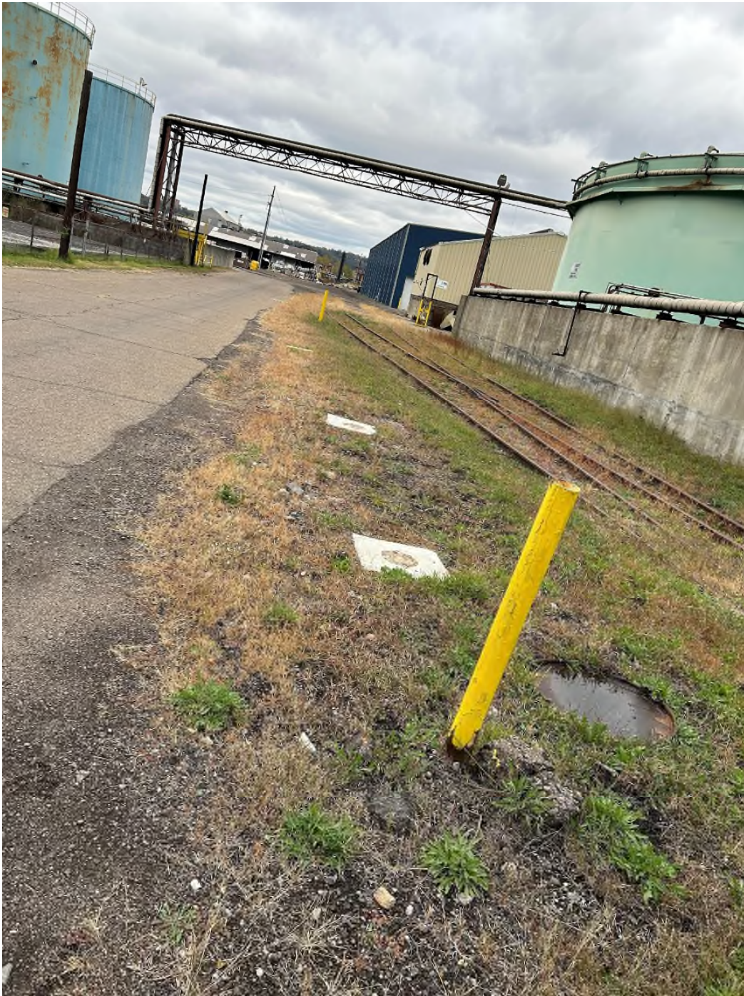
Figure 8: Looking north from the south end of the former plant. Flush mounted monitoring well cluster (R-222D, R-222I, R-222S) as well R-313 are in the foreground. Fresh appearance of concrete indicate recency of the flush mounts on the ground.
