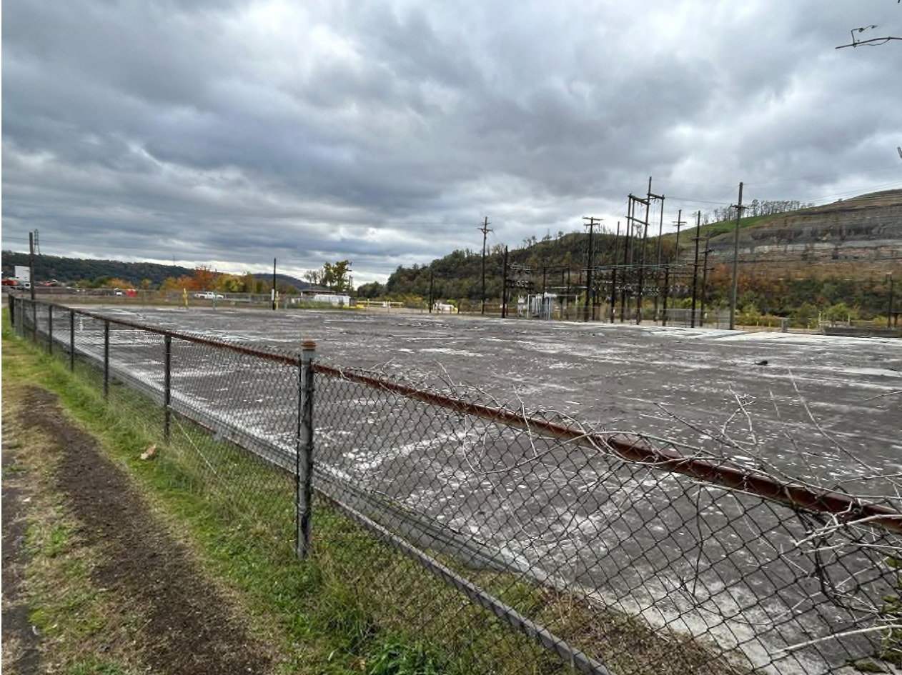
Figure 7: Looking southwest at the former aeration basins.
