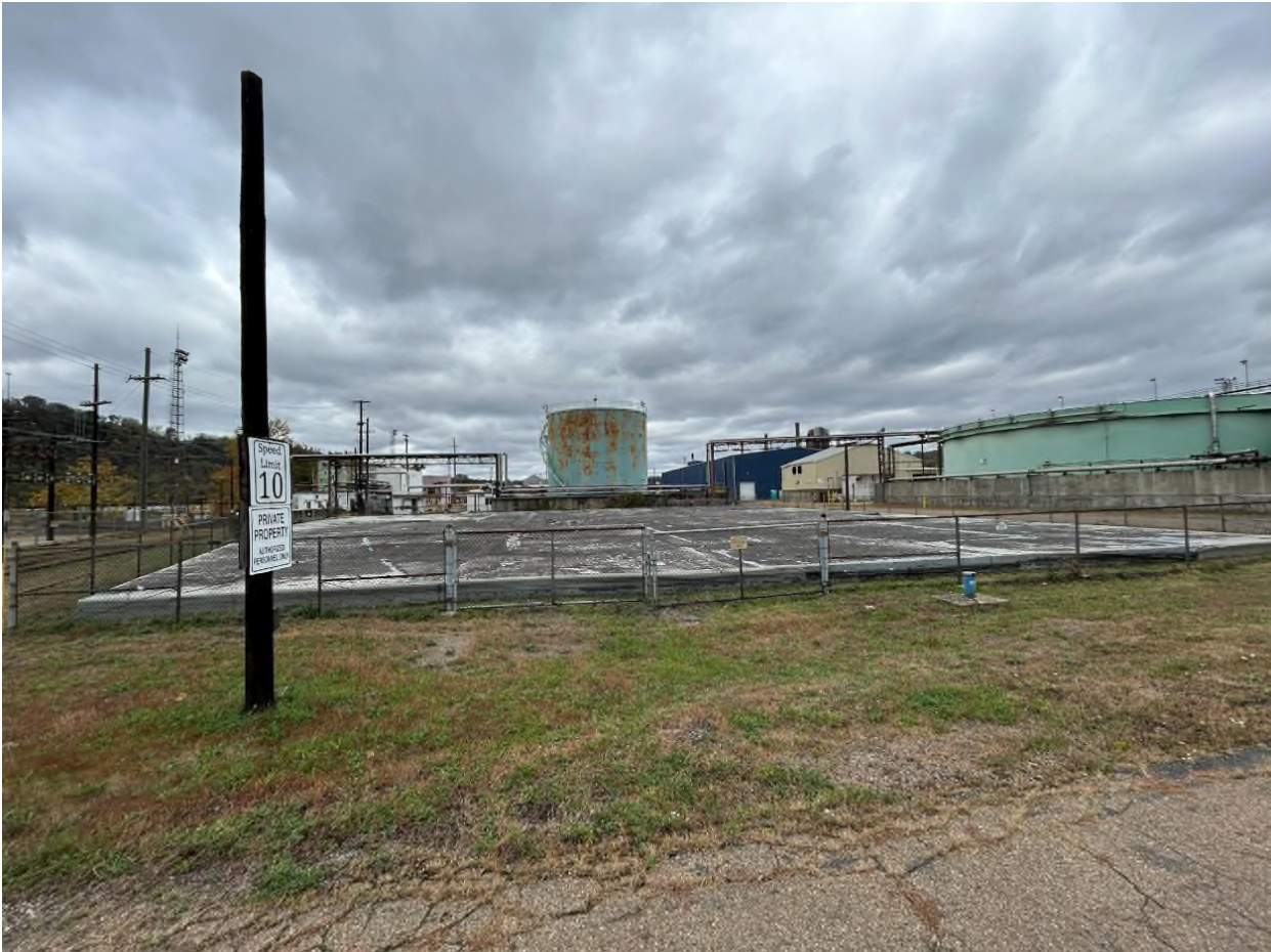
Figure 9: Looking north with the former aeration basins.
