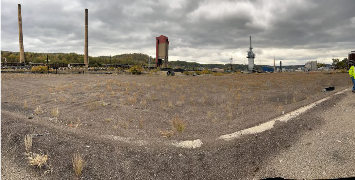
Figure 6: An open surface area of the former plant covered with what appears to be clean fill (smokestacks and process towers of the former Mountain State Carbon site in the background).
