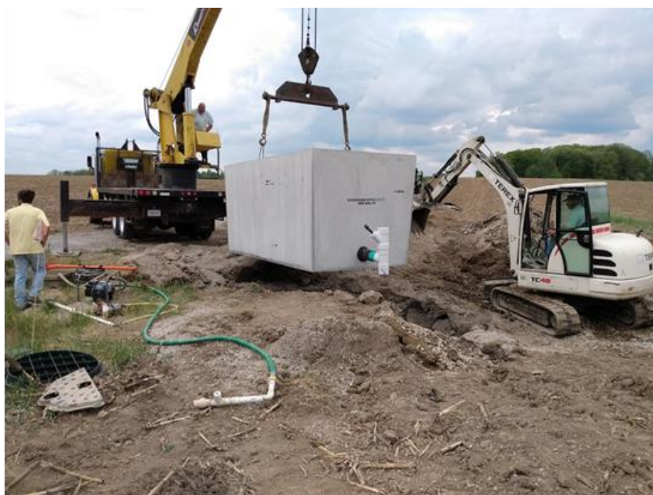
Installation of a P removal structure. Source: Chad Penn, USDA-ARS.
