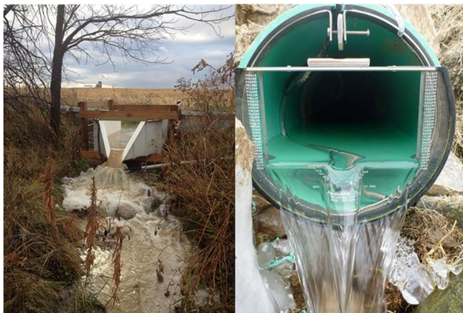
Example of edge-of-field surface (left) and subsurface (right) control volumes at data collection points. Source: Williams et al., 2016 .
