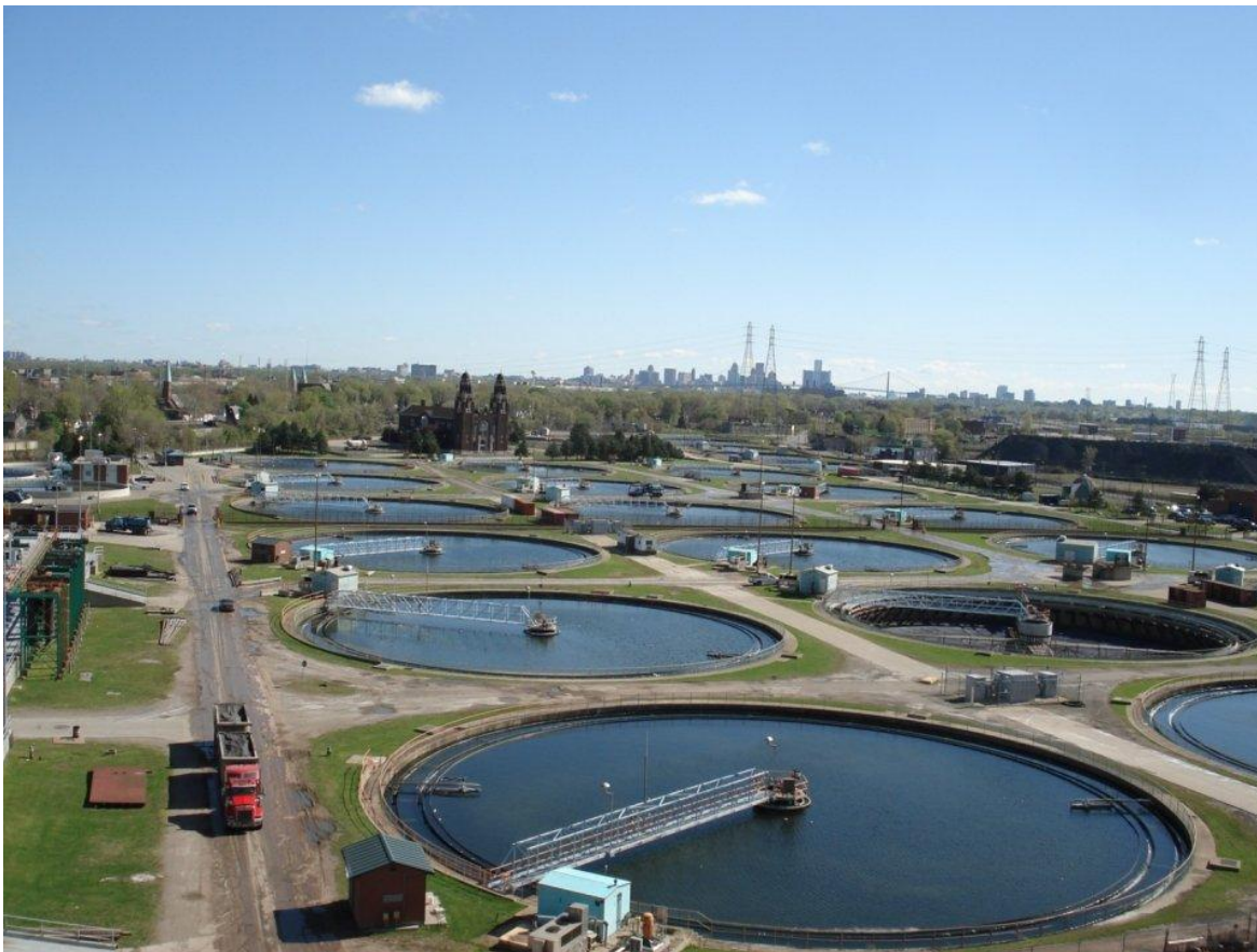
View of secondary clarifiers at the Great Lakes Water Authority's Water Resource Recovery Facility. Source: Michigan EGLE.
