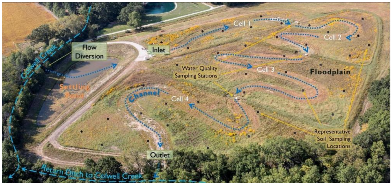
Aerial image of a phosphorus optimal wetland that shows the direction of water being diverted through the constructed wetland. Source: USACE.
