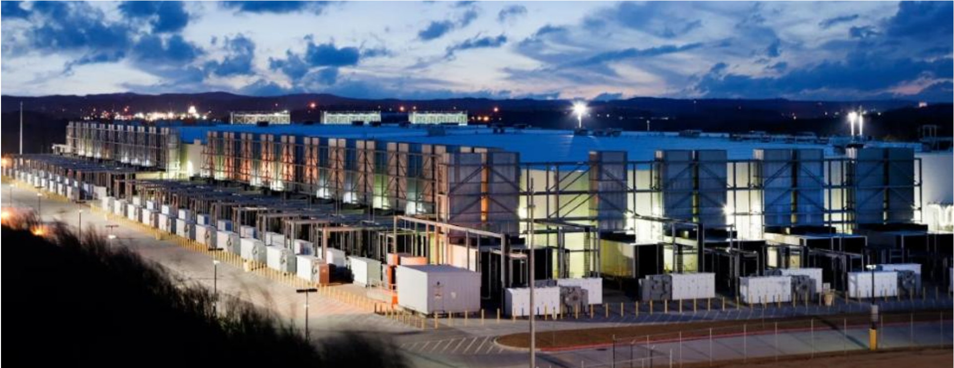
Google Data Center Douglas County, GA ~1 mgd reclaimed water
