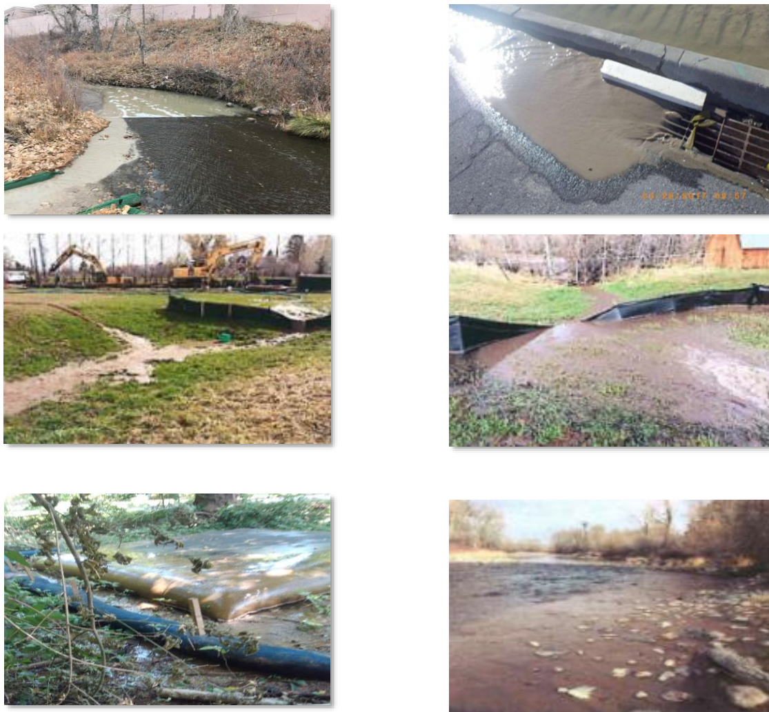
Figure 1. Photos depicting dewatering discharges from permitted construction sites.
