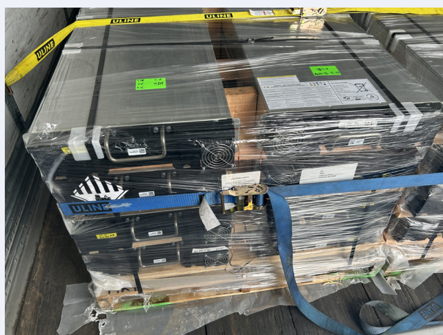
De-energized batteries packaged and ready to be sent for recycling
