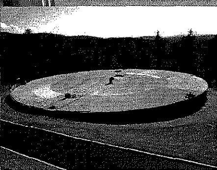
Finished Water Clearwell
