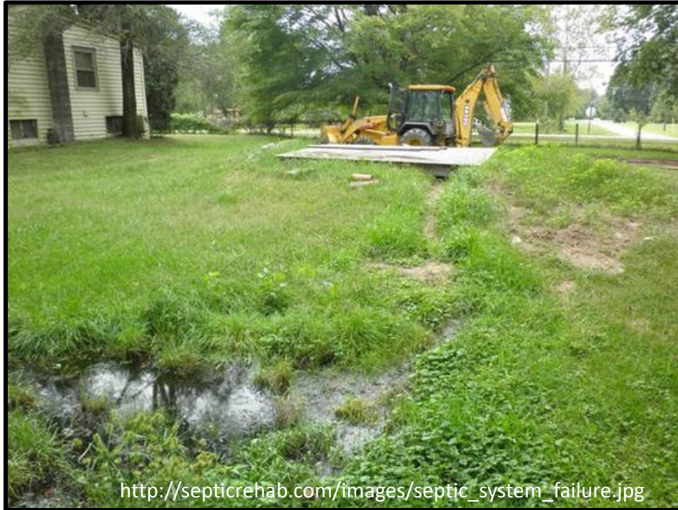
Failing septic system
