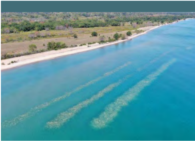
Aerial view of fully installed submerged rubble ridges at Illinois Beach State Park. Photo credit: US Army Corps of Engineers
