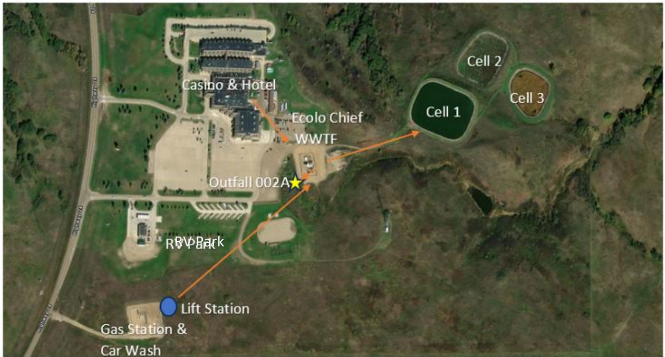
Figure 2. Overview of Prairie Knights Casino WWTF
