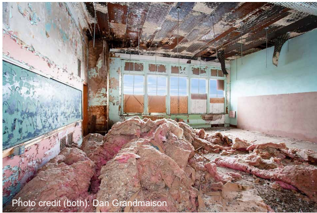
Photo credit (both): Dan Grandmaison Historic 3 rd floor classroom, future apartment
