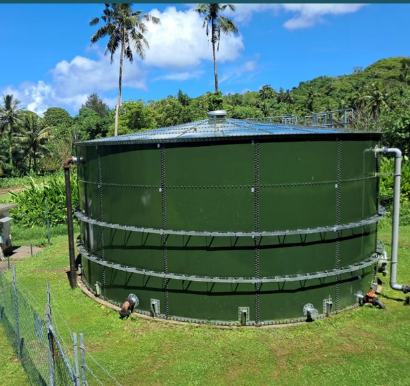
The newly installed water storage tank near Pava'ia'i village
