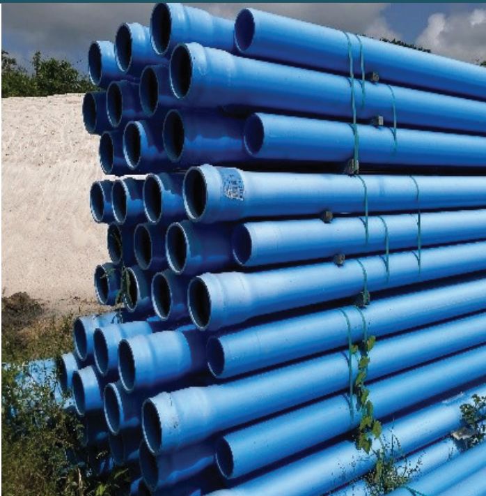
PVC pipe ready for installation by WAPA in the Campo Rico neighborhood
