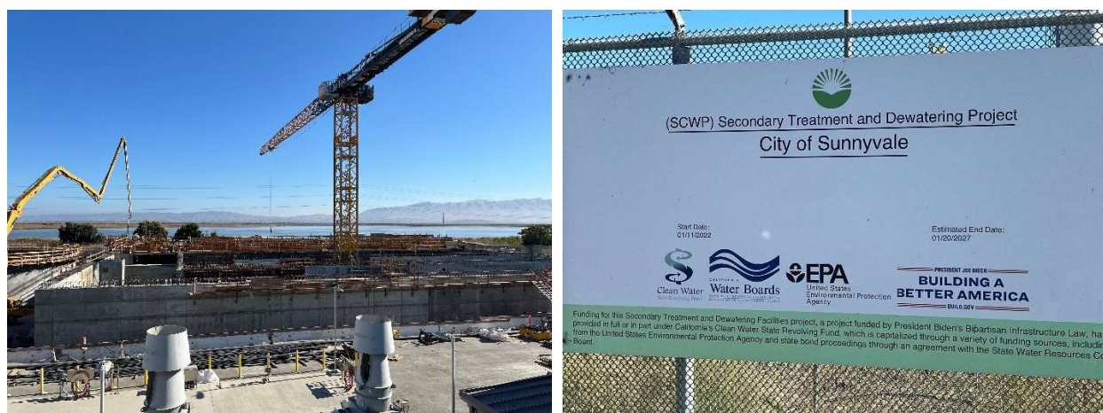
(Left) Construction cranes working over the Sunnyvale Project. (Right) A privacy fence along the edge of the site with the entrance sign that includes information about the EPA points of contact. (EPA OIG images)
