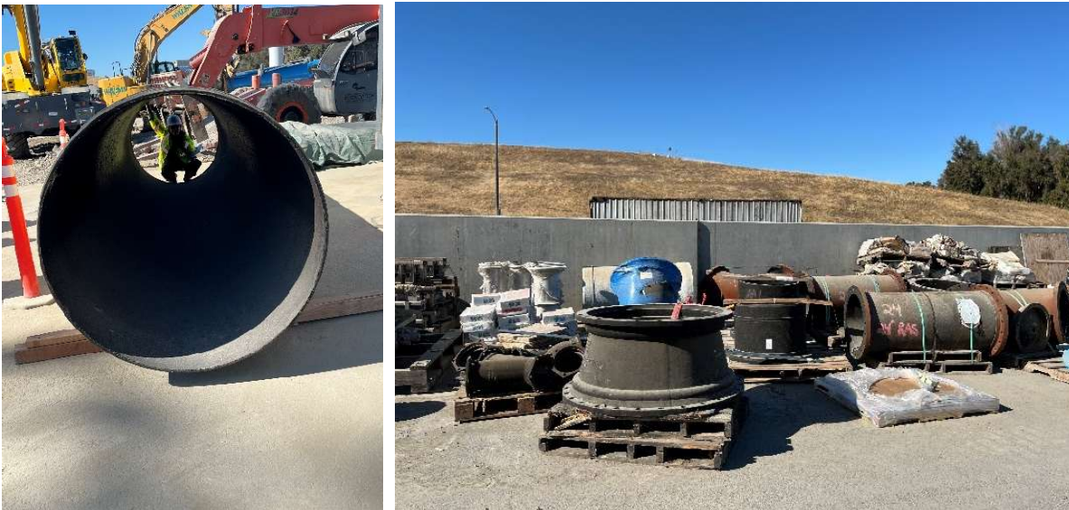
(Left) Large ductile iron pipe at the Sunnyvale Project site. (Right) Various iron and steel products waiting for installation. (EPA OIG images)
