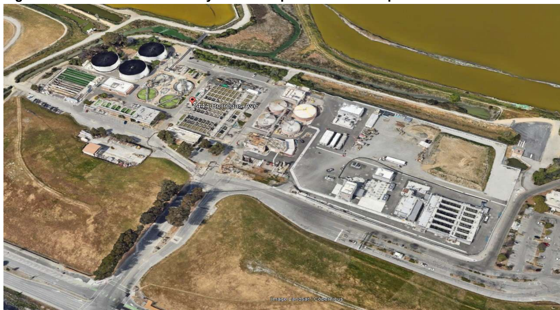
Figure 1: Aerial view of the Sunnyvale water pollution control plant
