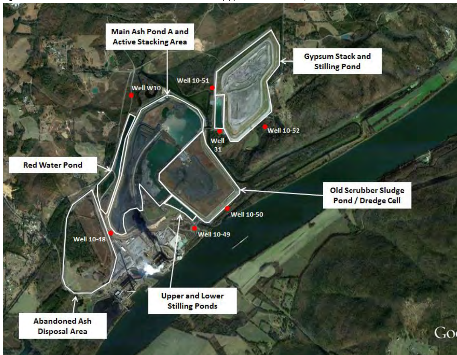
Figure 12-1: Groundwater wells at Widows Creek Fossil Plant (approximate locations)
