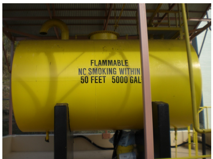
5000 gallon diesel fuel tank
