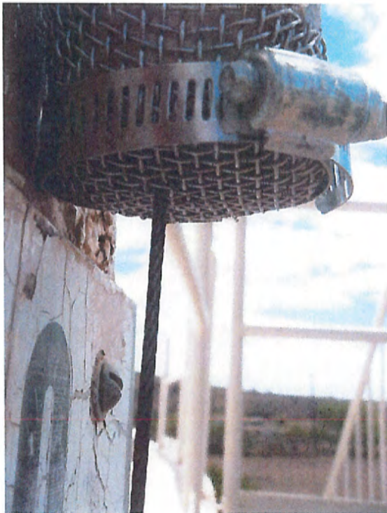
Photo 6: Halawa Tank S-2 – Water level cable pipe screened (CLOSEUP).
