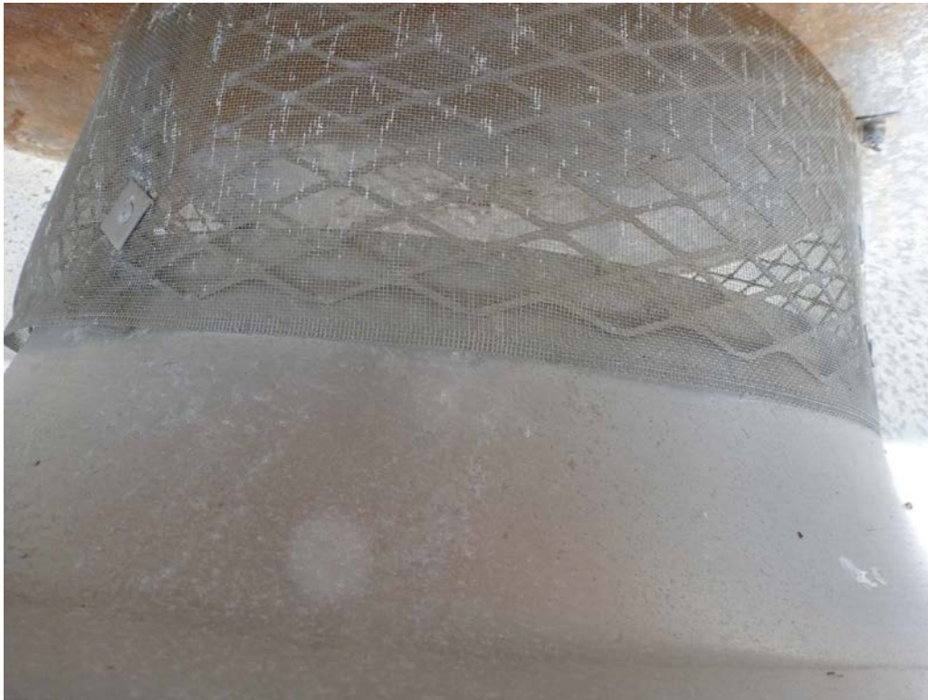
Tank 327: Secure loose bottom edge of roof vent screen.
