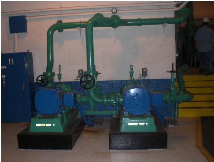
Red Hill Booster Pumps 1 & 2, 500 GPM each
