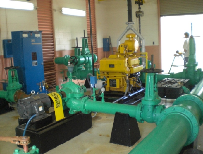
Left: Manana Booster Pump Station has 2 booster pumps (green) & 1 diesel pump for fire protection (yellow) Right: 300 gallon diesel fuel tank at Manana Booster Pump Station
