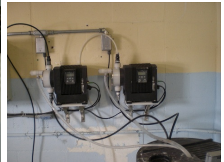
Fluoride injector pumps
