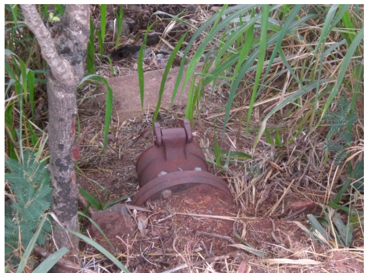
Overflow outlet pipe with flapper valve
