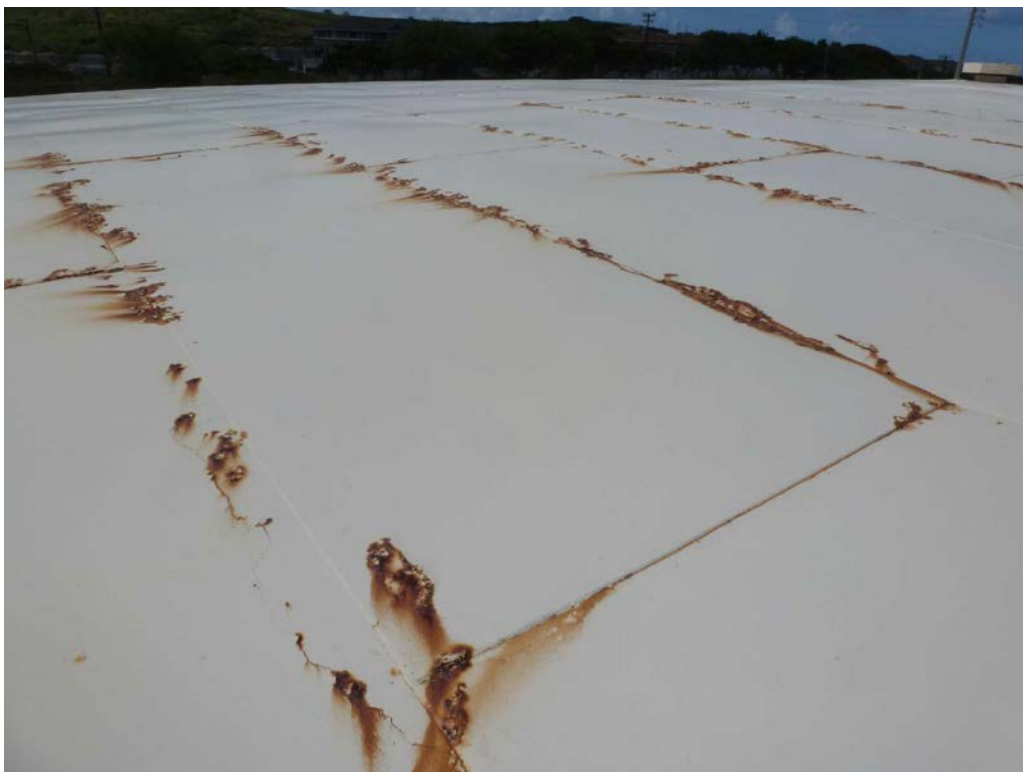
Halawa Tank S-1 : Rust observed on the roof should be addressed.
