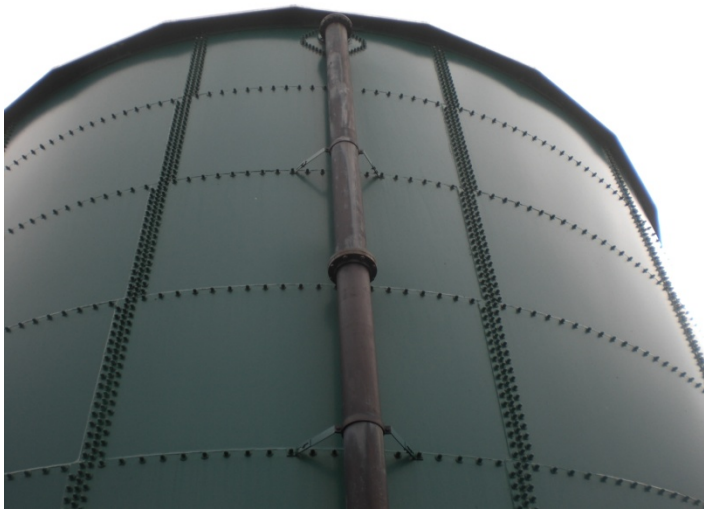
Red Hill Storage Tank, 250,000 gallon, glass-lined steel
