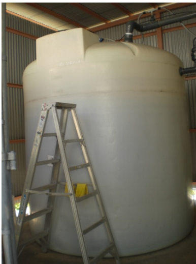
Sodium Hypochlorite Tank
