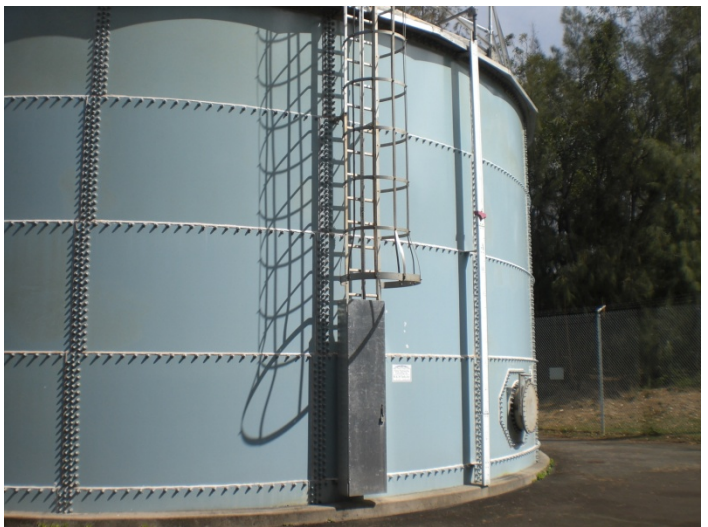
Access Hatch with rubber gasket
