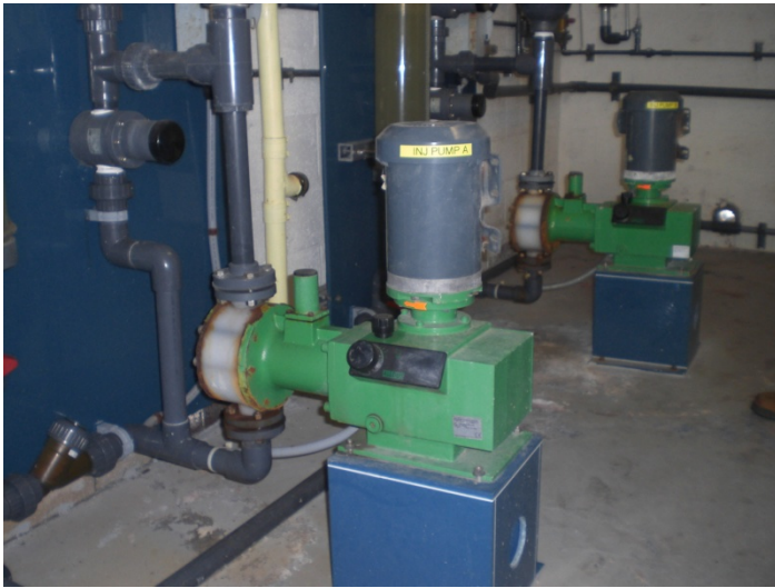
Sodium Hypochlorite injector pumps
