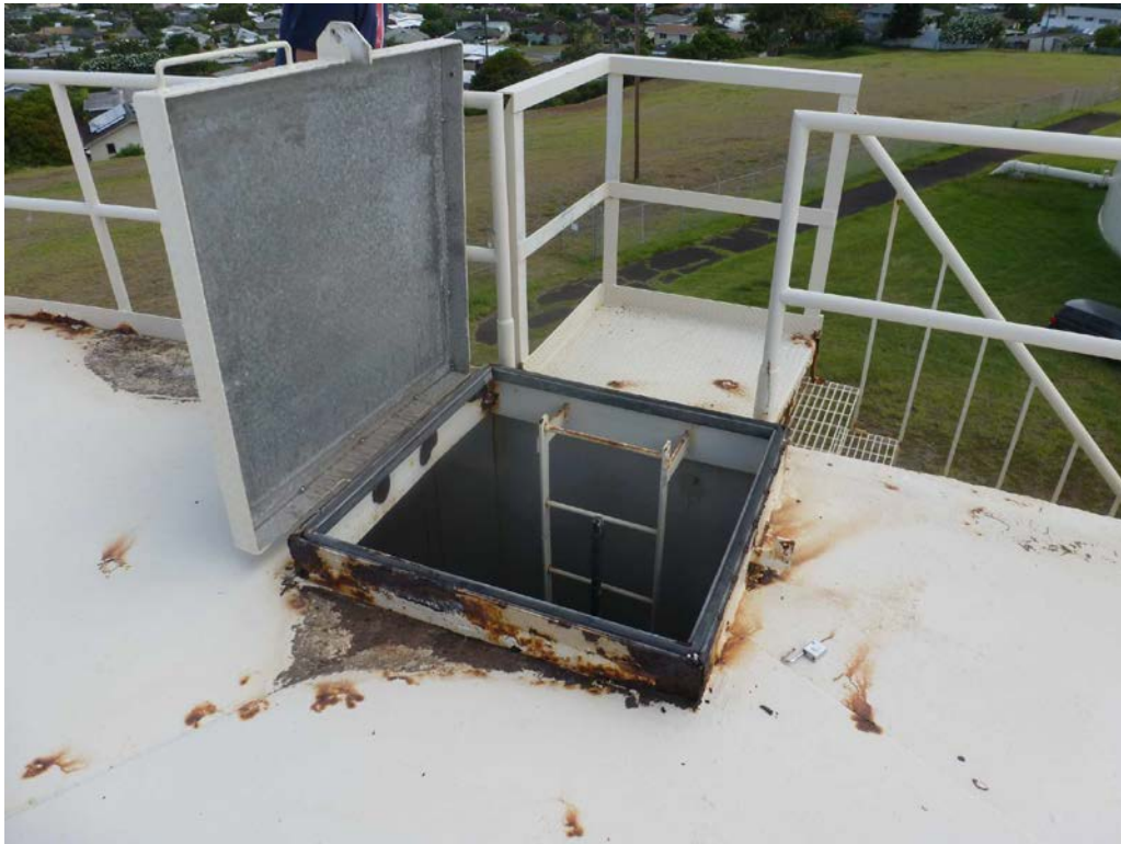
Halawa Tank S-1: Severe rust in the roof hatch has created holes in the raised steel curb providing an entryway for contaminants, insects and geckos. The openings should be repaired and sealed in the interim. The current project to reconstruct the roof hatch should be expedited.
