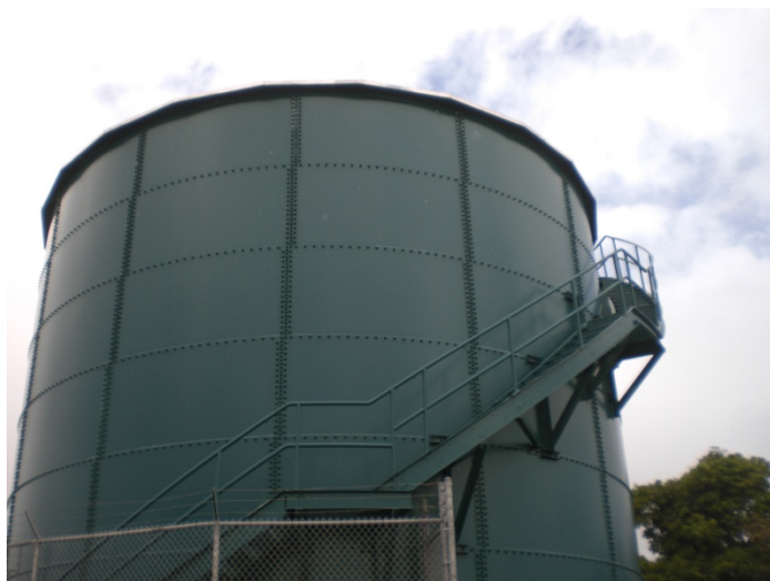
Red Hill Storage Tank, 250,000 gallon, glass-lined steel
