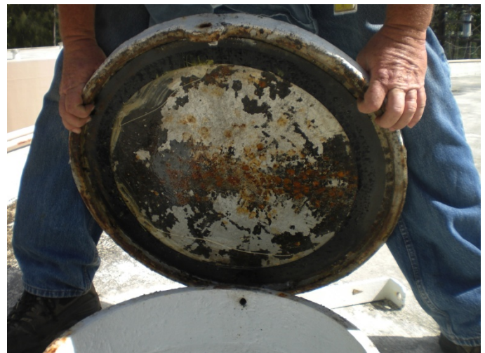
Access Hatch with rubber gasket
