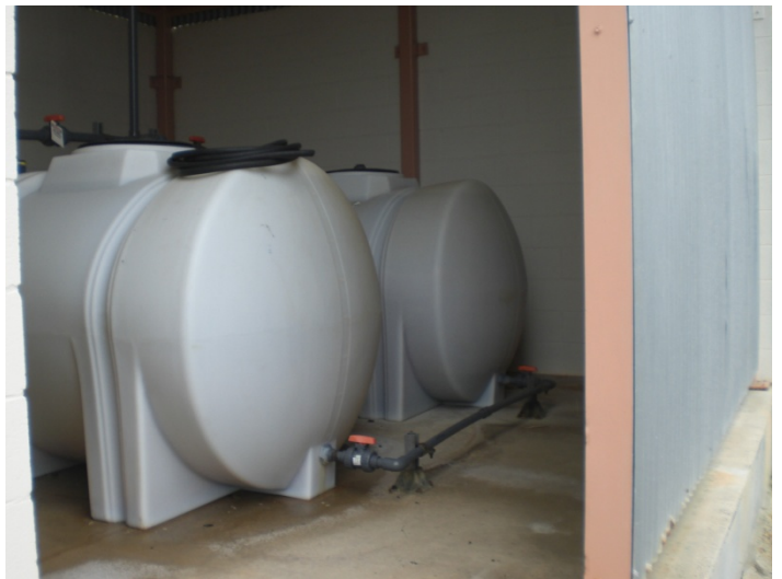
Sodium Hypochlorite Storage Tanks
