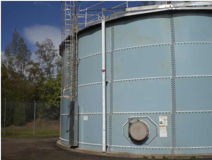
Storage Tank S-327, 140,000 gallons, Glass-lined steel, Camp Smith
