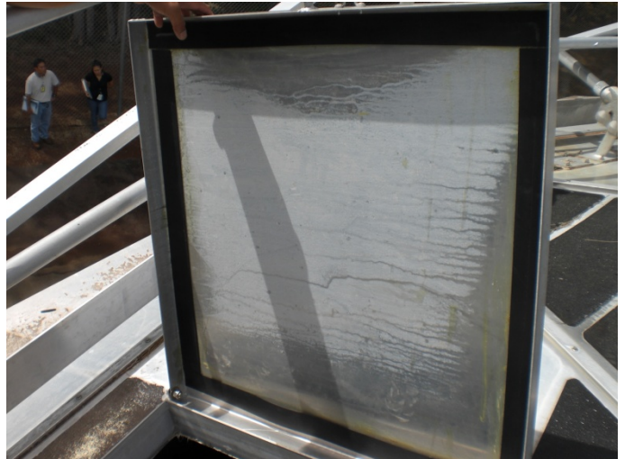
Access Hatch with rubber gasket
