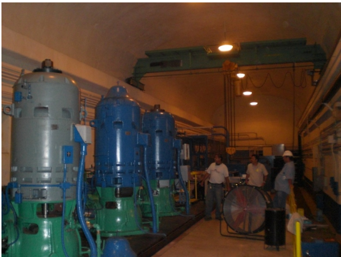
Red Hill Pump Room, 4 pumps @ 6,500 GPM each
