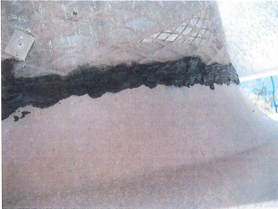
Photo 1: Camp Smith Tank S-327 – Secured bottom edge of vent screen
