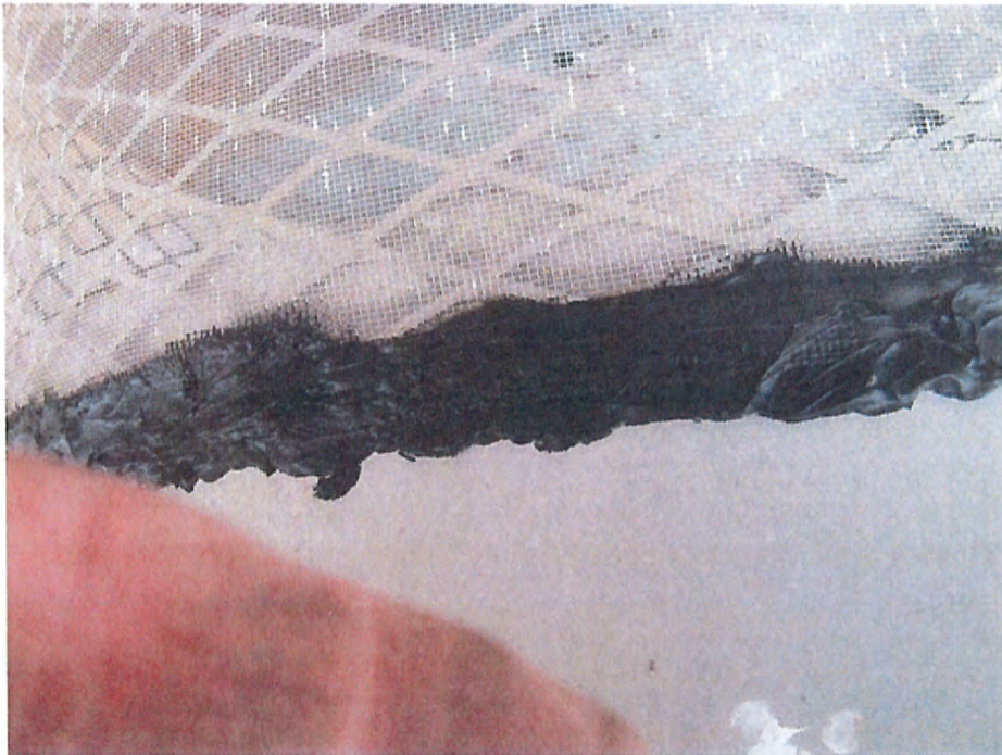
Photo 2: Camp Smith Tank S-327 – Secured bottom edge of vent screen (CLOSEUP).
