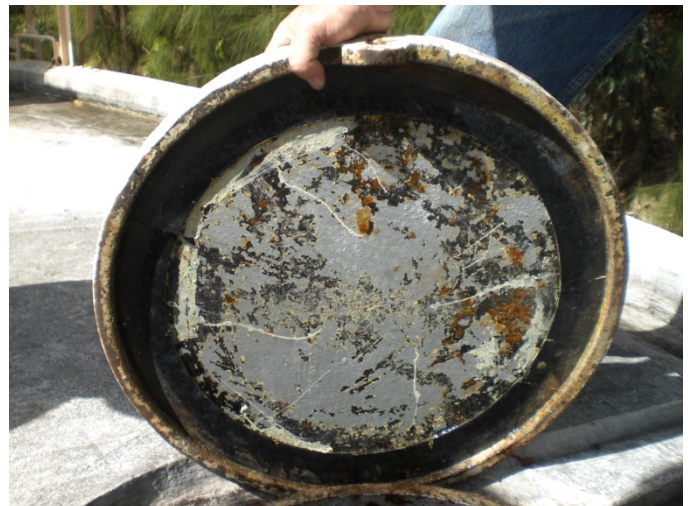
Access Hatch with rubber gasket
