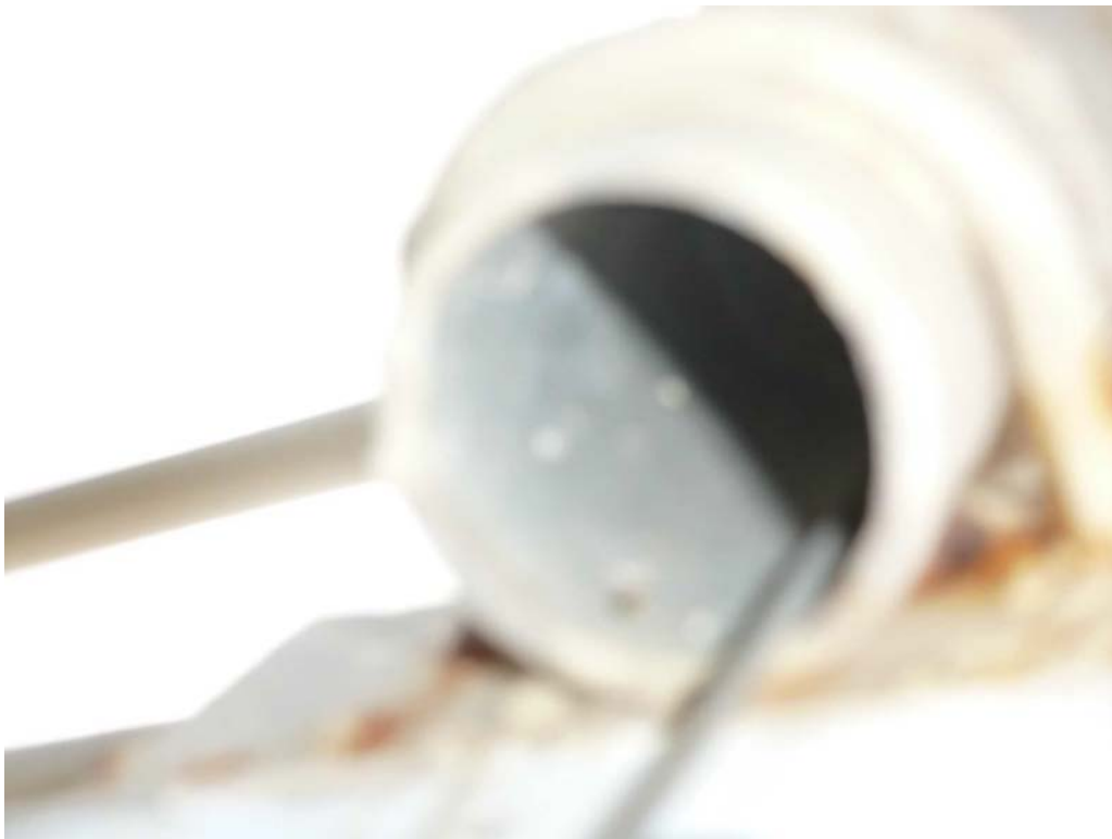
Halawa Tank S-2: Plug open end of water level cable pipe.
