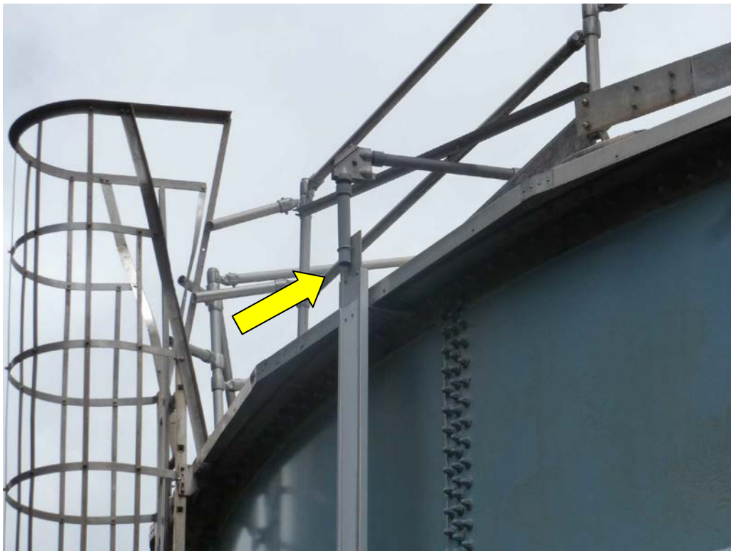
Tank 327: Plug open end of water level cable pipe.
