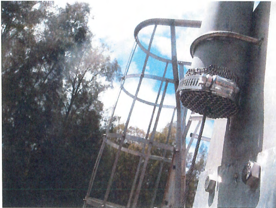
Photo 3: Camp Smith Tank S-327 – Water level cable pipe screened
