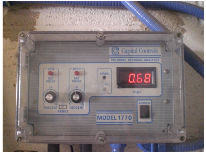
Chlorine Residual Analyzer
