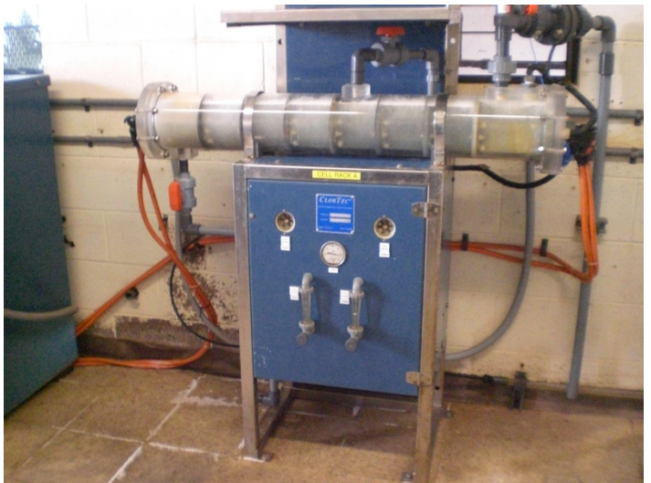
ClorTec sodium hypochlorite generation system (2 units)
