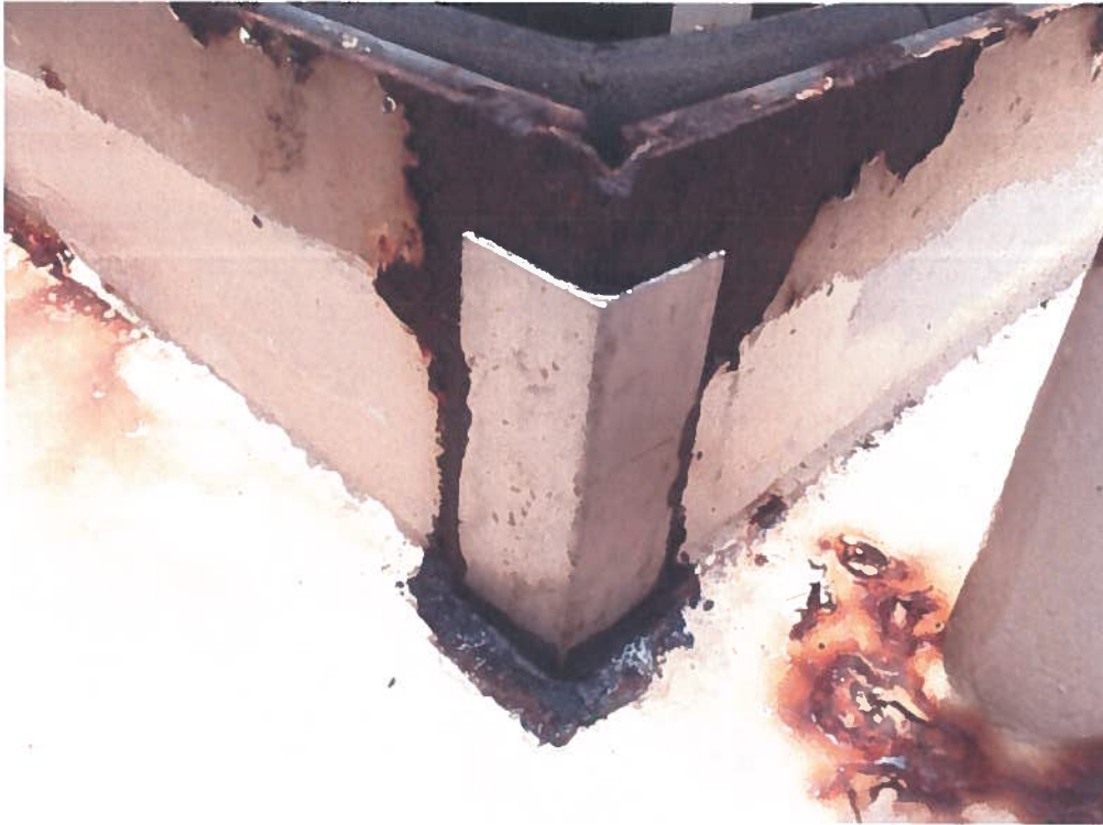
Photo 3: Close up view of patch on opposite corner of hatch
