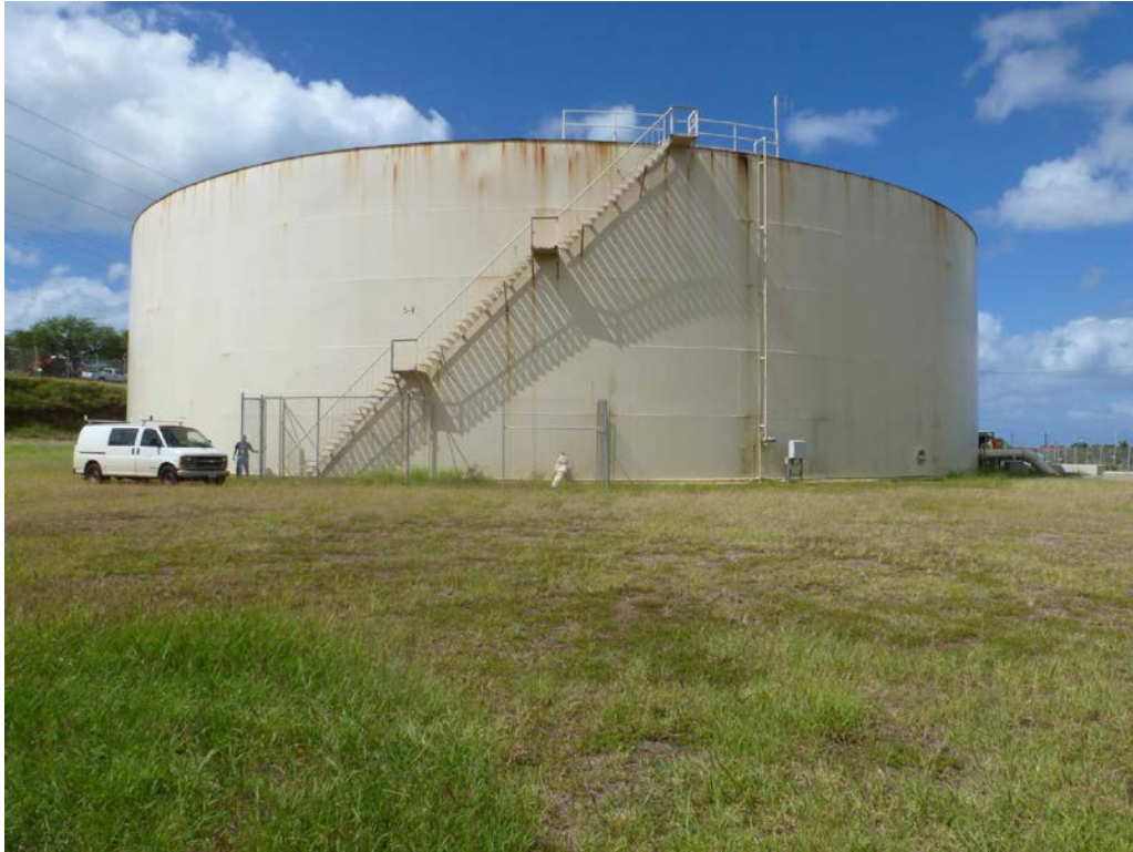
Halawa Tank S-1 : The rust observed on the exterior tank walls near the roofline, on the roof surface and in the steel stairway should be addressed before the rust progresses further.
