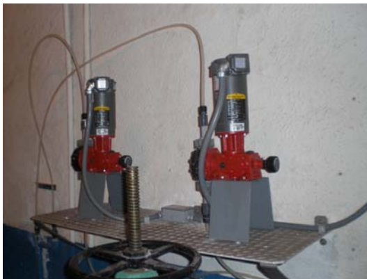
Fluoride injector pumps
