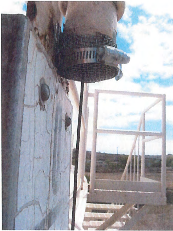
Photo 5: Halawa Tank S-2 – Water level cable pipe screened
